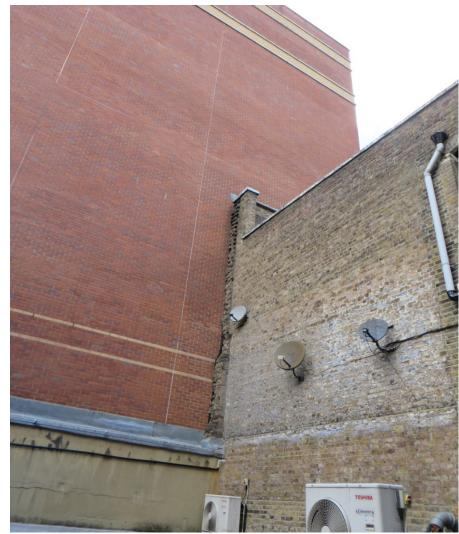
View lookinh north east fron first floor level to junction of rear of 125 Clerkenwell Road and 127 Clerkenwell Road. Note poor quality of brickwork, especially snapped headers at junction of two properties, and abscence of architectural features of any merit.
