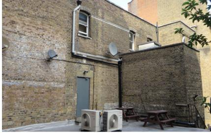
View looking north-east at first floor level to the rear of 125 Clerkenwell Road. Note lack of features, poor quality of brickwork, haphazard rear extensions and drainage runs.
