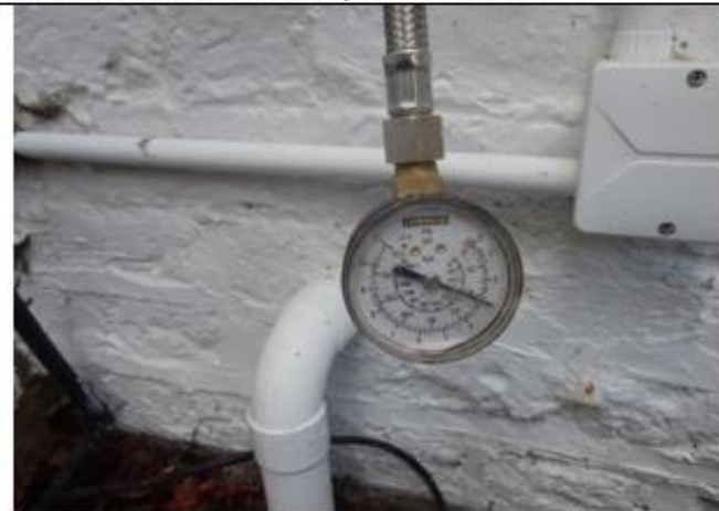
5. Mains water pressure test.
