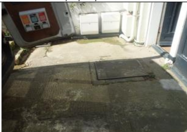
17. Front surface area.
