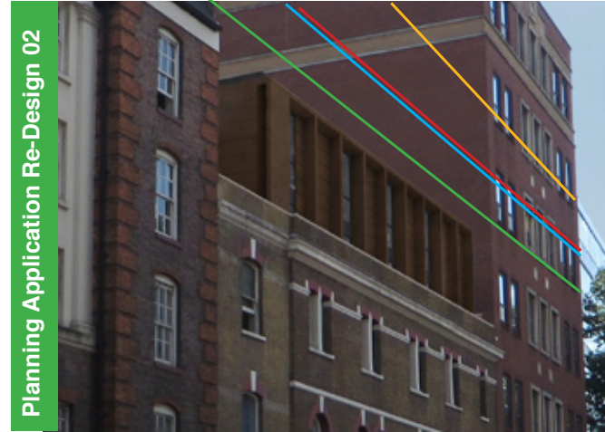
Scheme option submitted to council on 19th of April 2016 following advice from council that a modern approach would be appropriate. Further design amendments were requested by the council and agreed at the meeting at the council offices on 11th of July 2016. The attached revised skim was prepared following this meeting.
