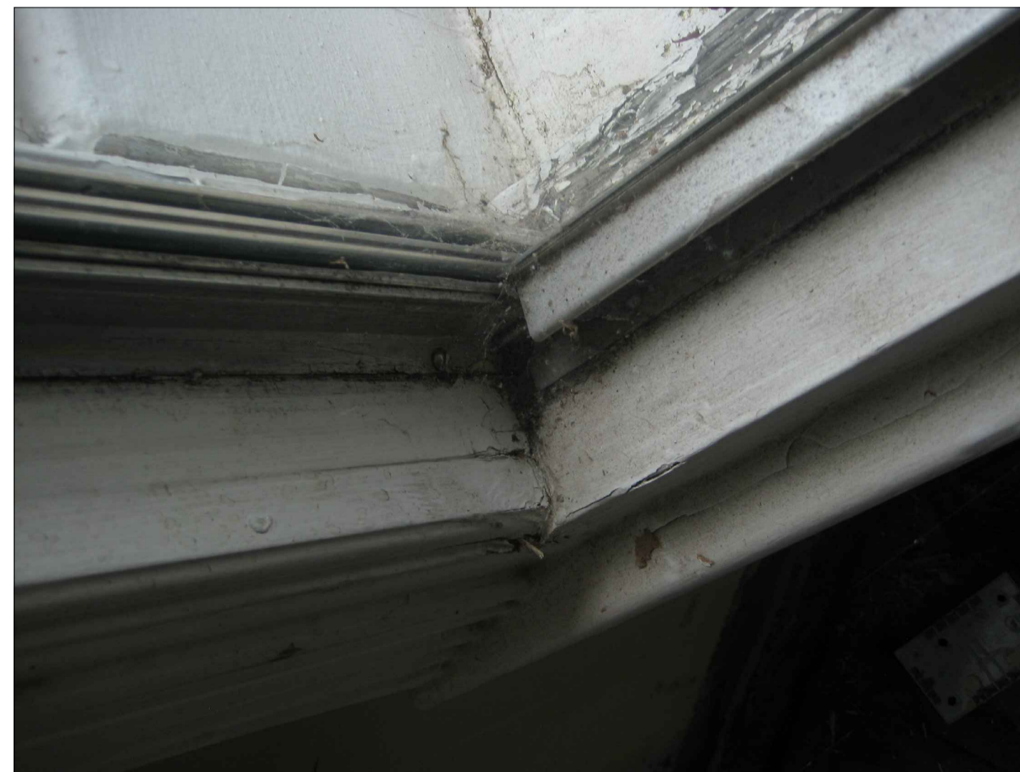
FIRST FLOOR WINDOWS GENERAL CONDITION OF REPAIR
