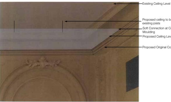
Proposed ceiling to be hung from existing joists Soft Connection at Cornice Lower Moulding Proposed Ceiling Level
