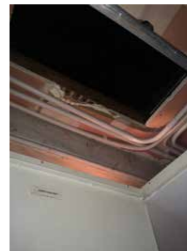
Current Access Hatch to Bedroom 2.
