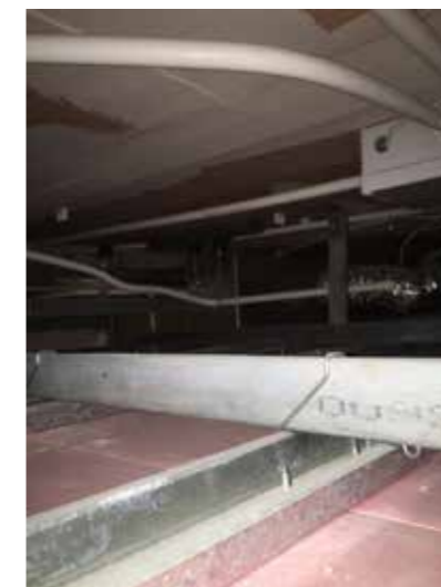
Current Dining Room Non Original Ceiling Void.
