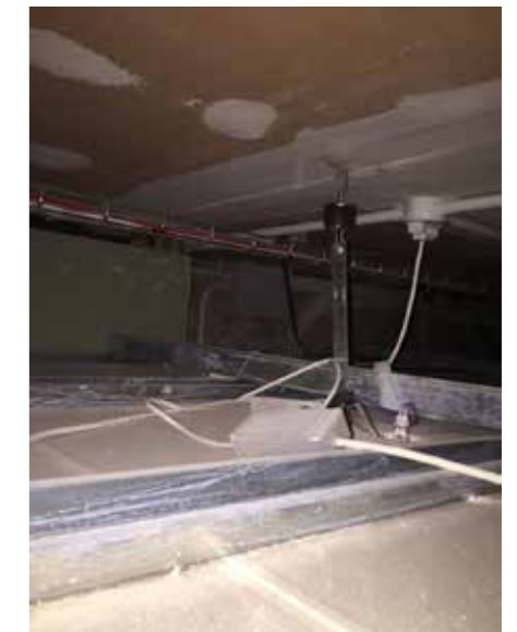
Current Ceiling Void to Kitchen.
