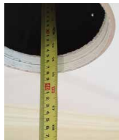
Current Master Ensuite Non Original Double Plasterboard Ceiling.
