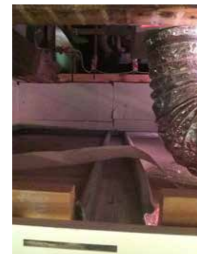
Current Ceiling Void to Bedroom 3 Ensuite.
