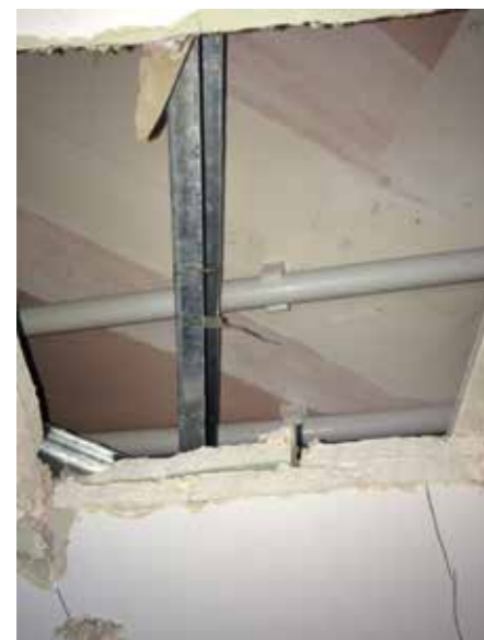
Current Secondary Hallway Non Original Ceiling Void.
