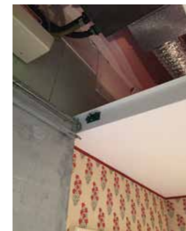
Current Master Dressing Room Non Original Ceiling Void.
