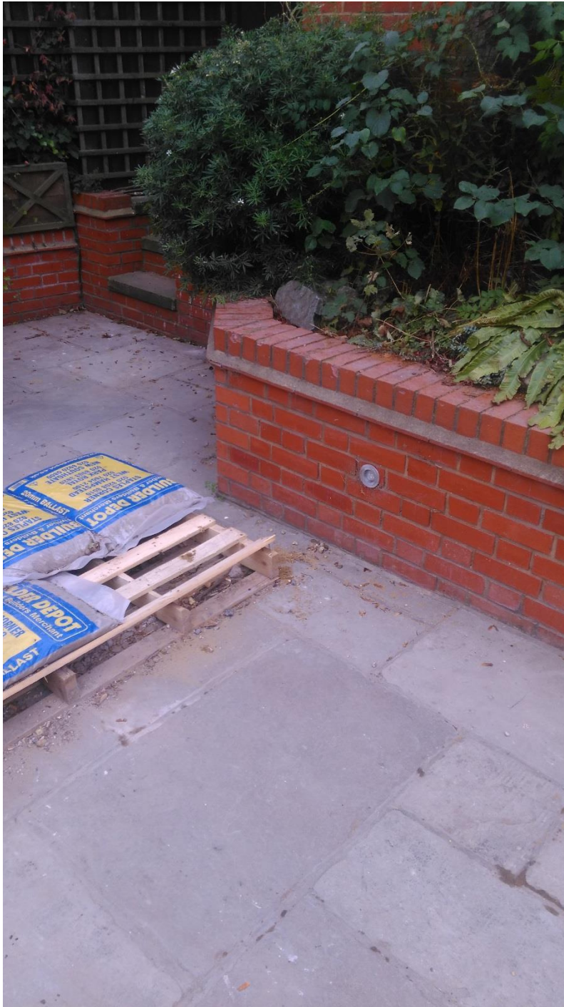
(Above) The existing surface paving and retaining wall for raised flower bed
