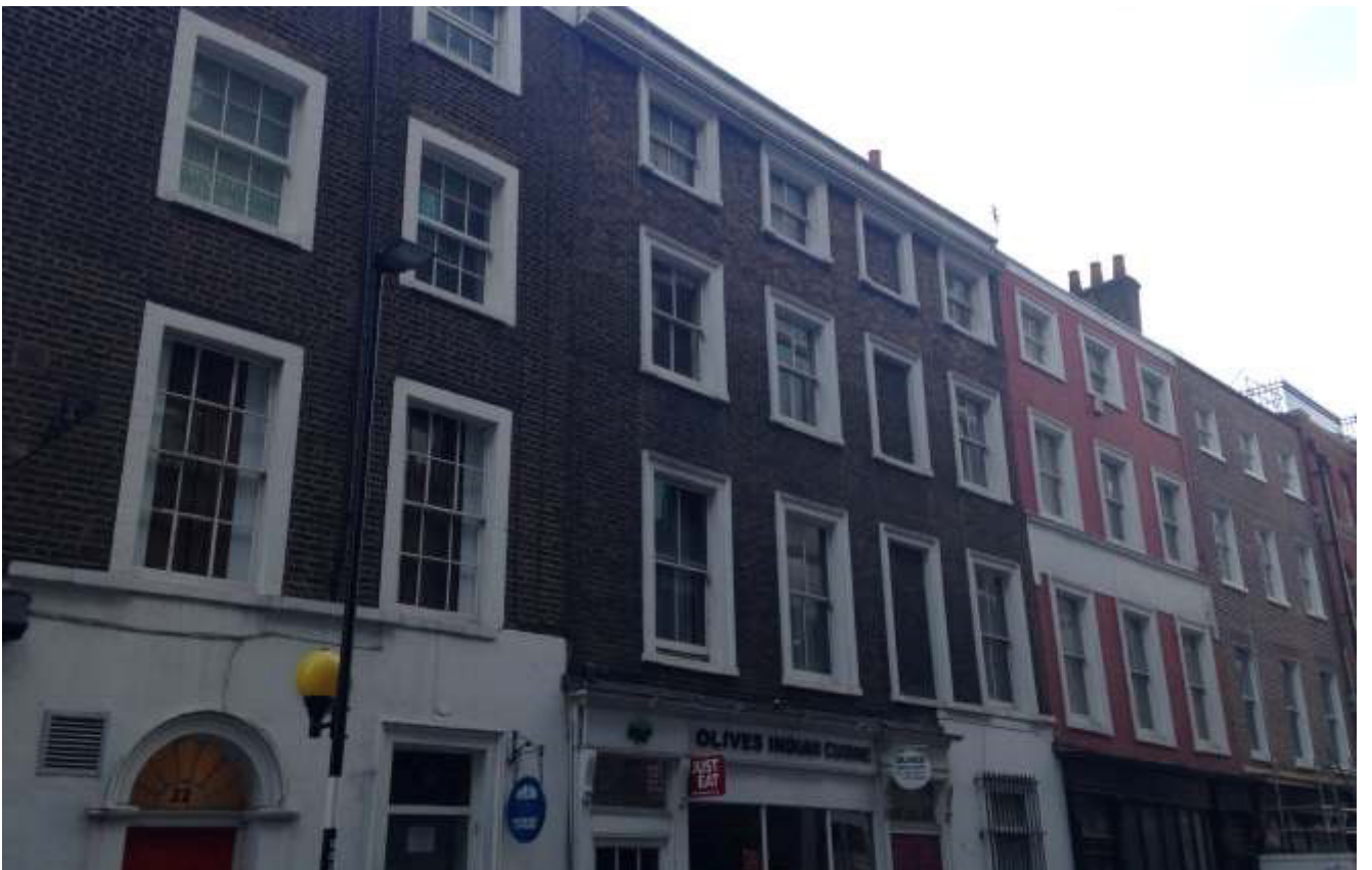
Front view of existing double glazed windows on Cleveland street
