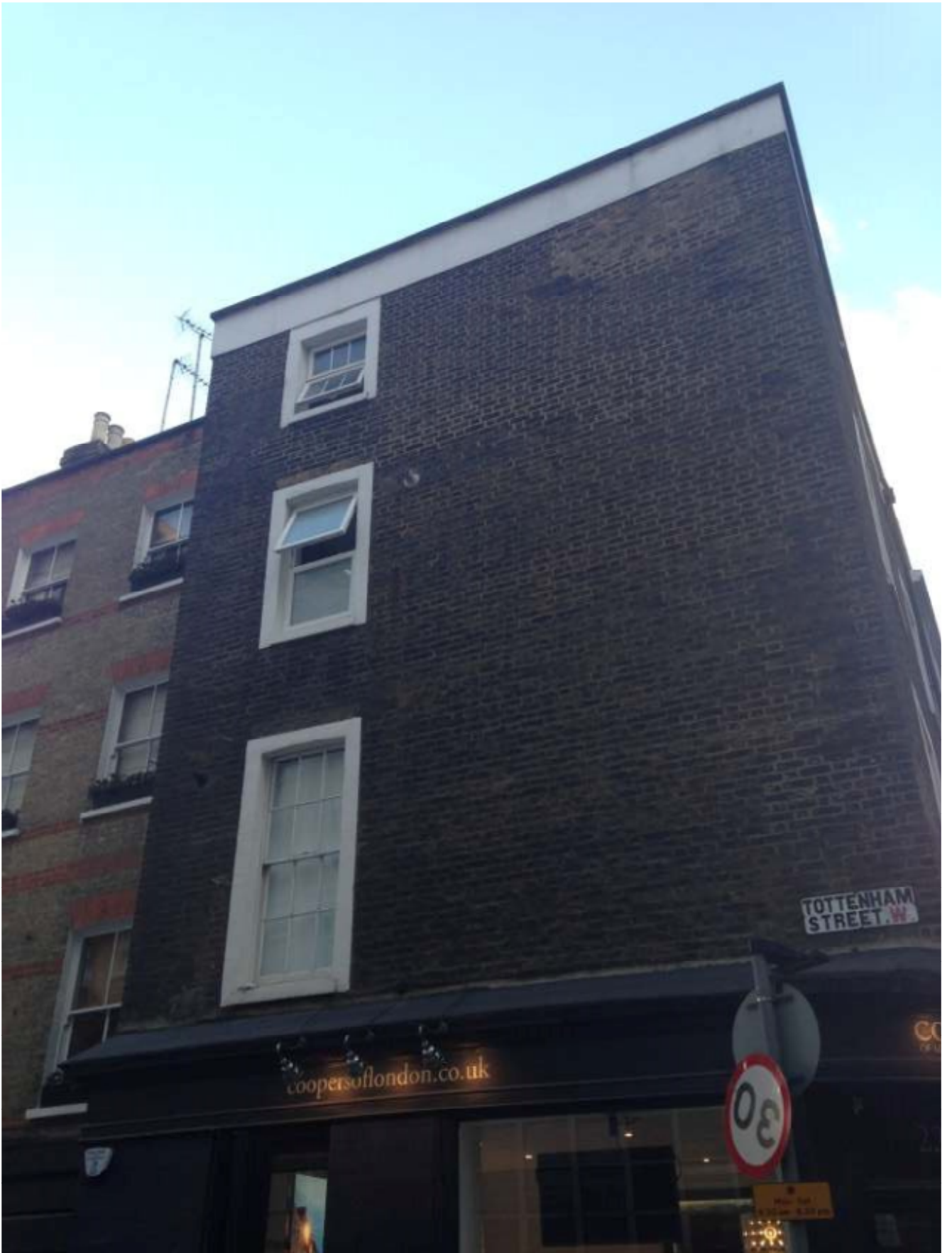
Existing casement window in the bathroom on Tottenham street
