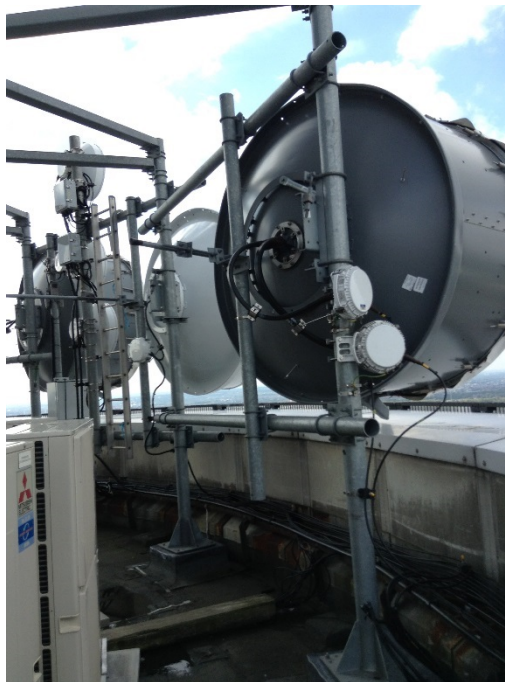
Photograph of the steelwork/antenna array to which the proposed antennas will be attached
