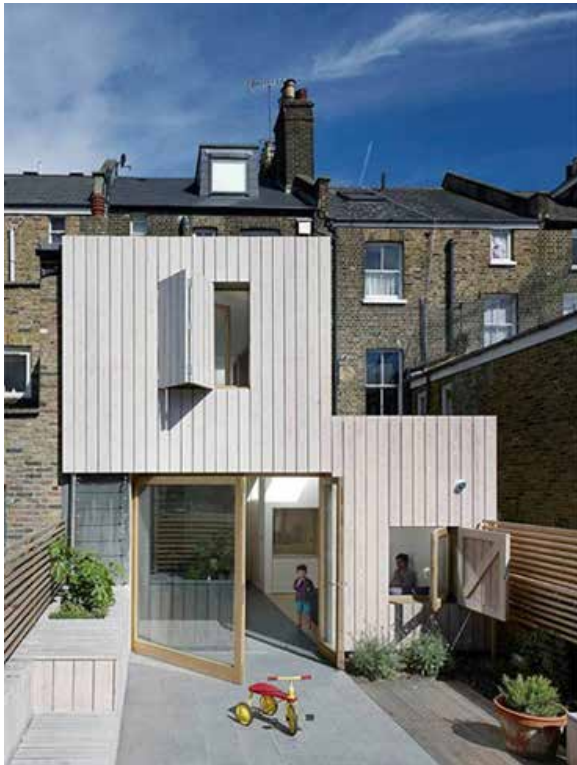
House extension in Camden with two distinct volumes
