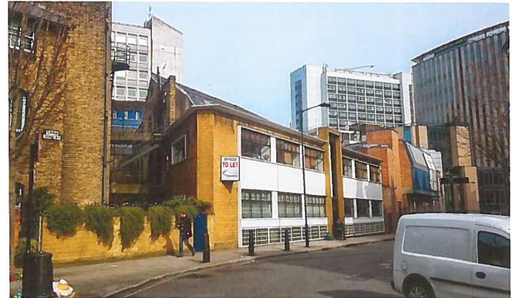
New GF entrance wall
