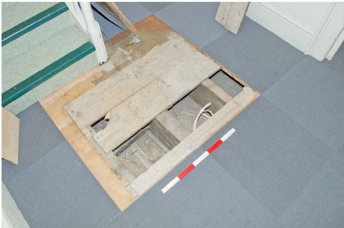
Floor structure of the second floor landing, looking south
