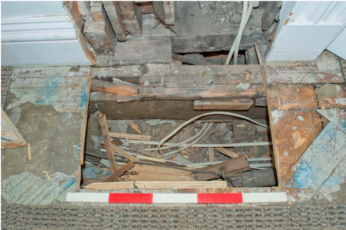
Structure of the first floor (front range), looking south-west
