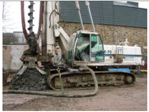
Photograph 2: Piling Rig CM-70
