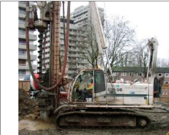
Photograph 1: Piling Rig CM-50
