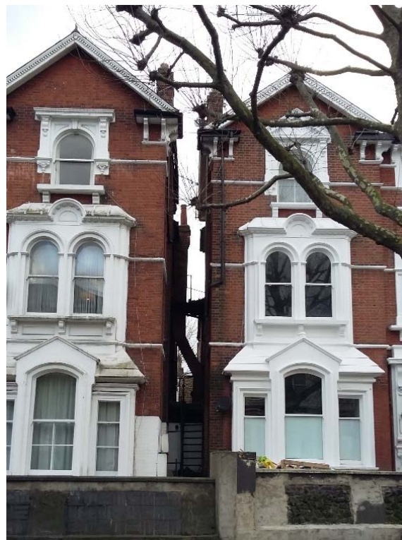
4 – Metal stair in between 129 & 131 West End Lane
