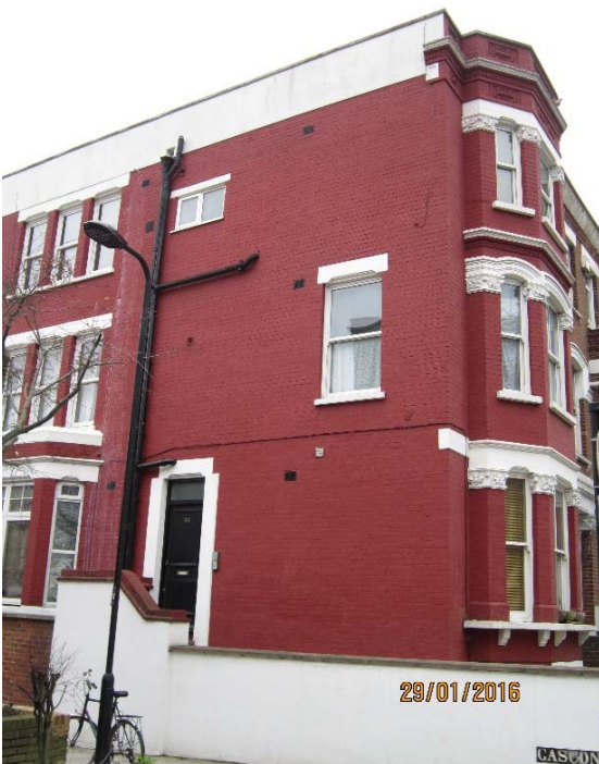
3 – Side access at the corner of West End Lane & Gascon Avenue
