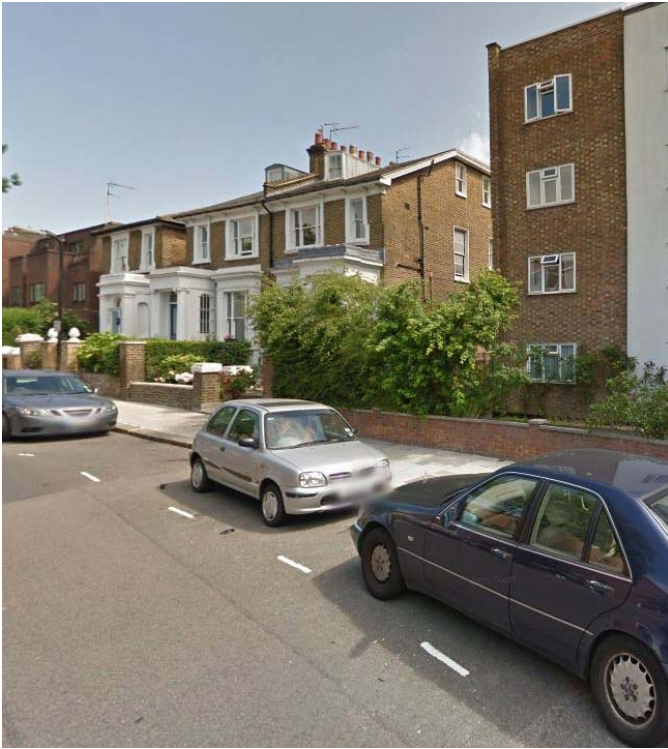
5 – Street view of the side elevation 1
