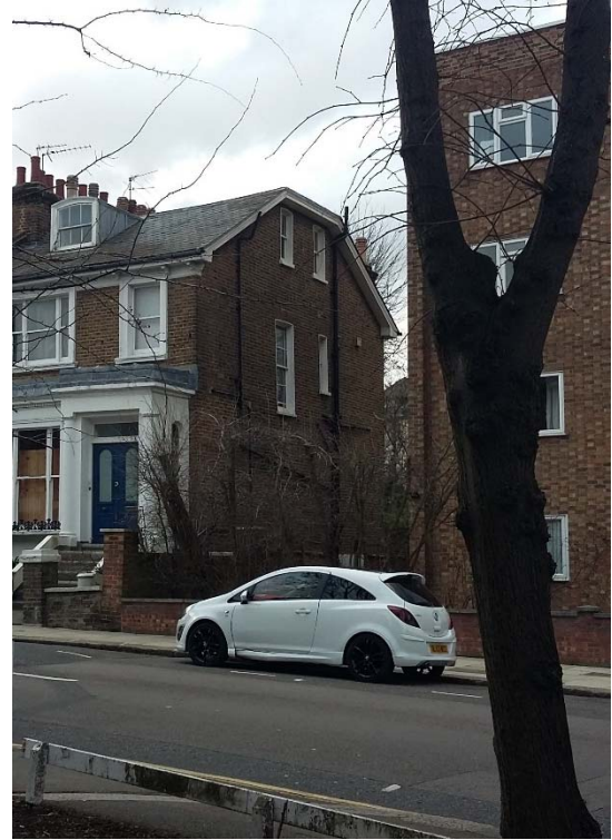
6 – Street view of the side elevation 2
