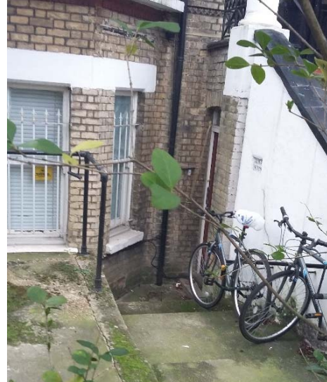
2 – Photograph of 56 West End Lane
