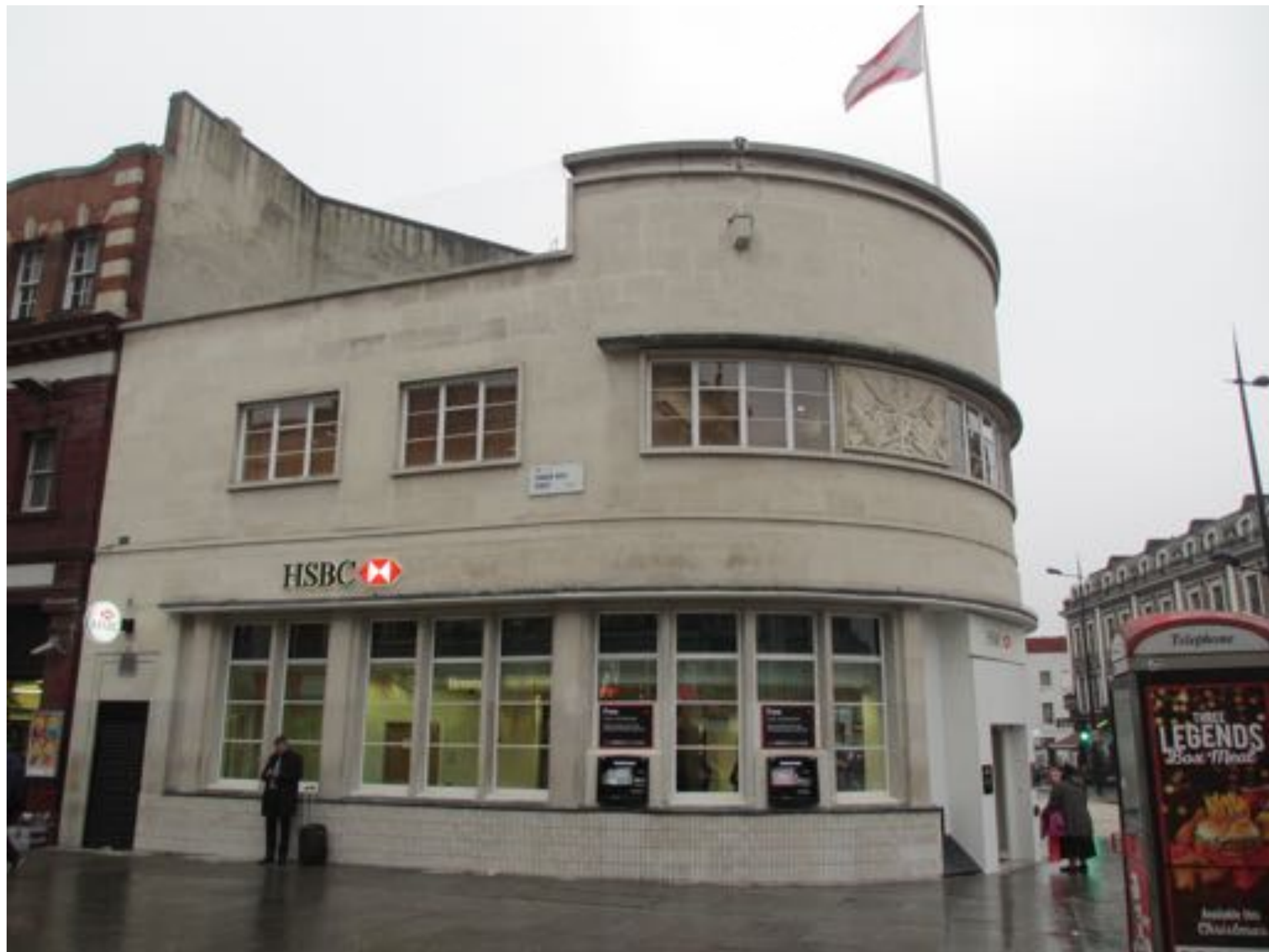
PHOTOGRAPH OF SIDE ELEVATION
