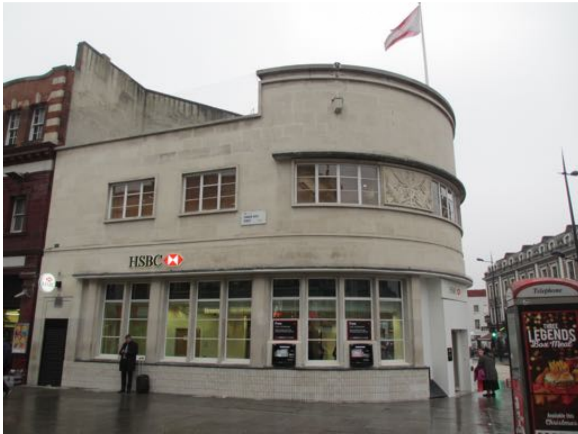
PHOTOGRAPH OF SIDE ELEVATION
