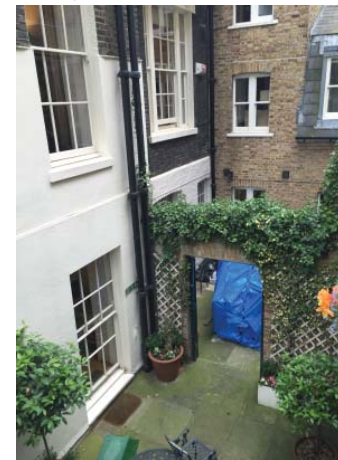
Looking down into the rear courtyard, No. 1 partially rendered at low level, the courtyard of No. 2 through arch.
