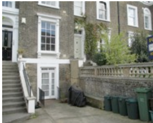
Existing forecourt showing concrete retaining dwarf wall to number 10
