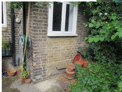
existing bricked up opening showing original door opening
