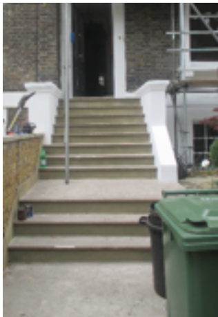
York stone staircase reference on neighbouring property
