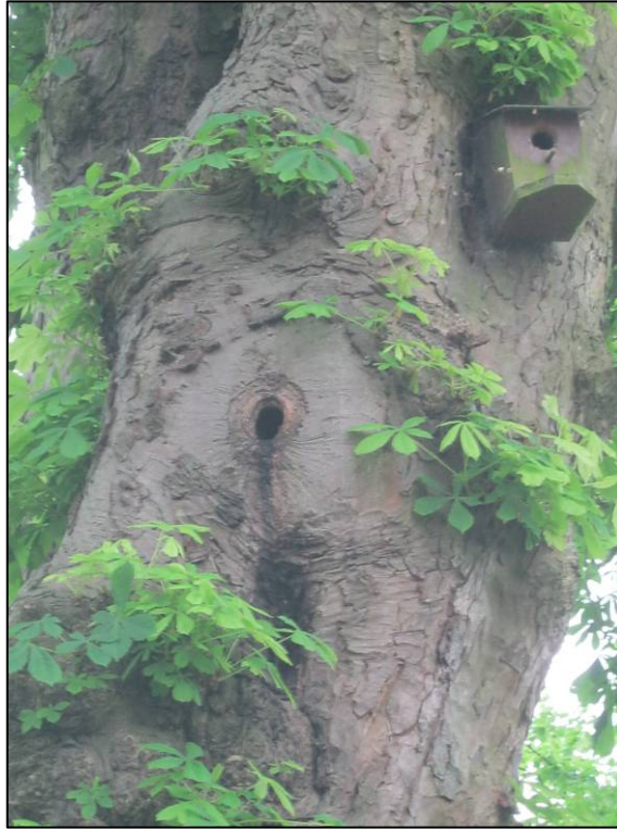
Fig 13 Hole in horse chestnut shown in Fig 12, with staining typical of bats.
