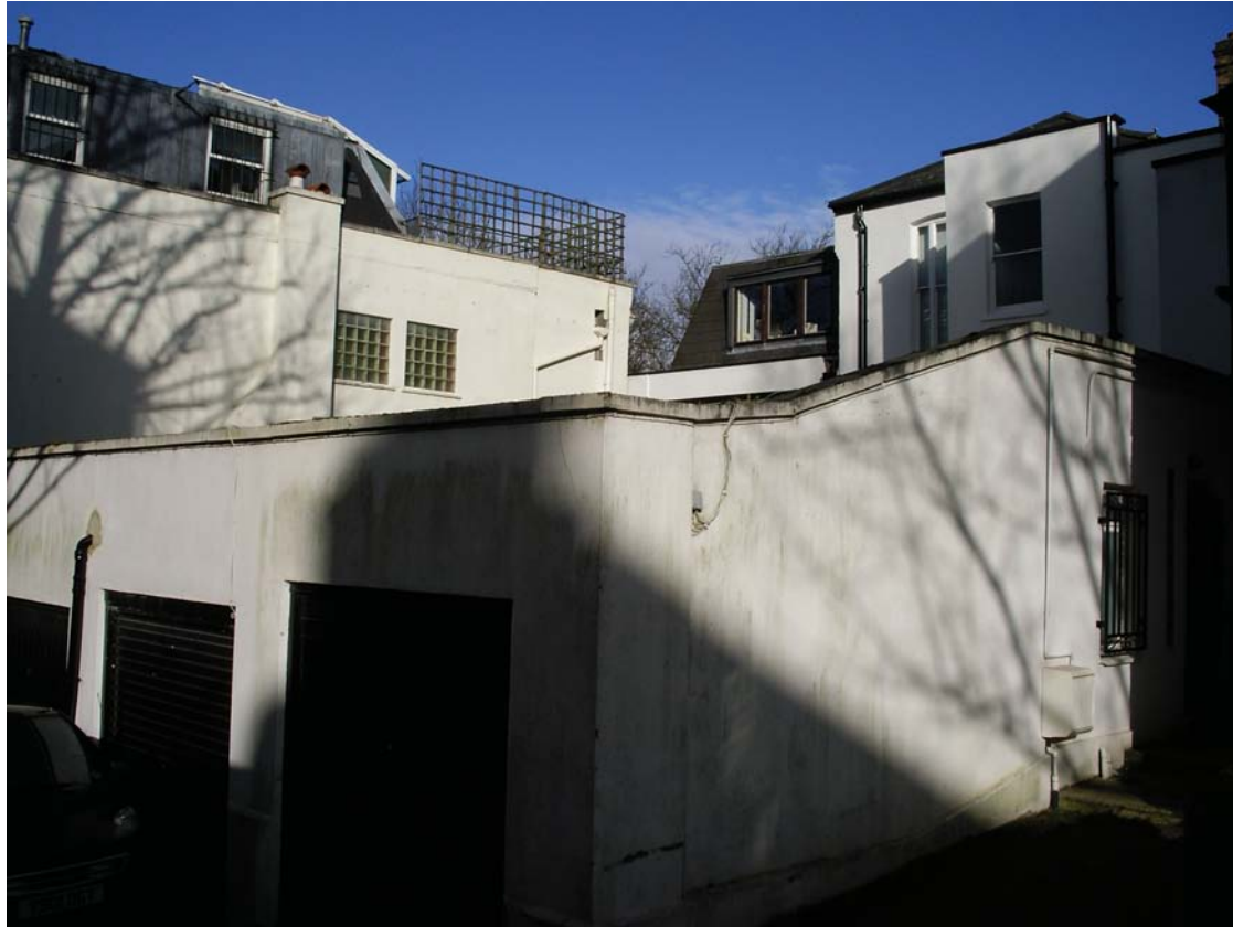
Rear view of Ladywell Court.
