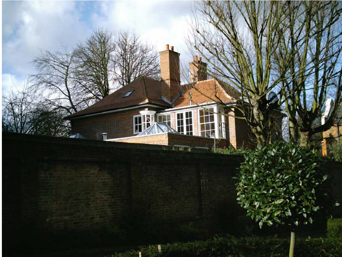
View of property opposite & 10ft. wall.
