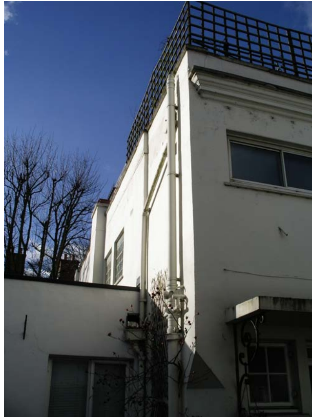
View of 10 Ladywell Court and adjoining apartment.
