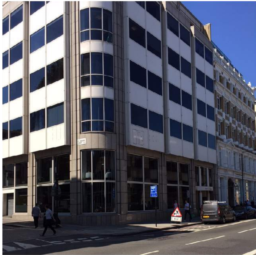
Figure 1.2: Existing Office Building / Application Site
