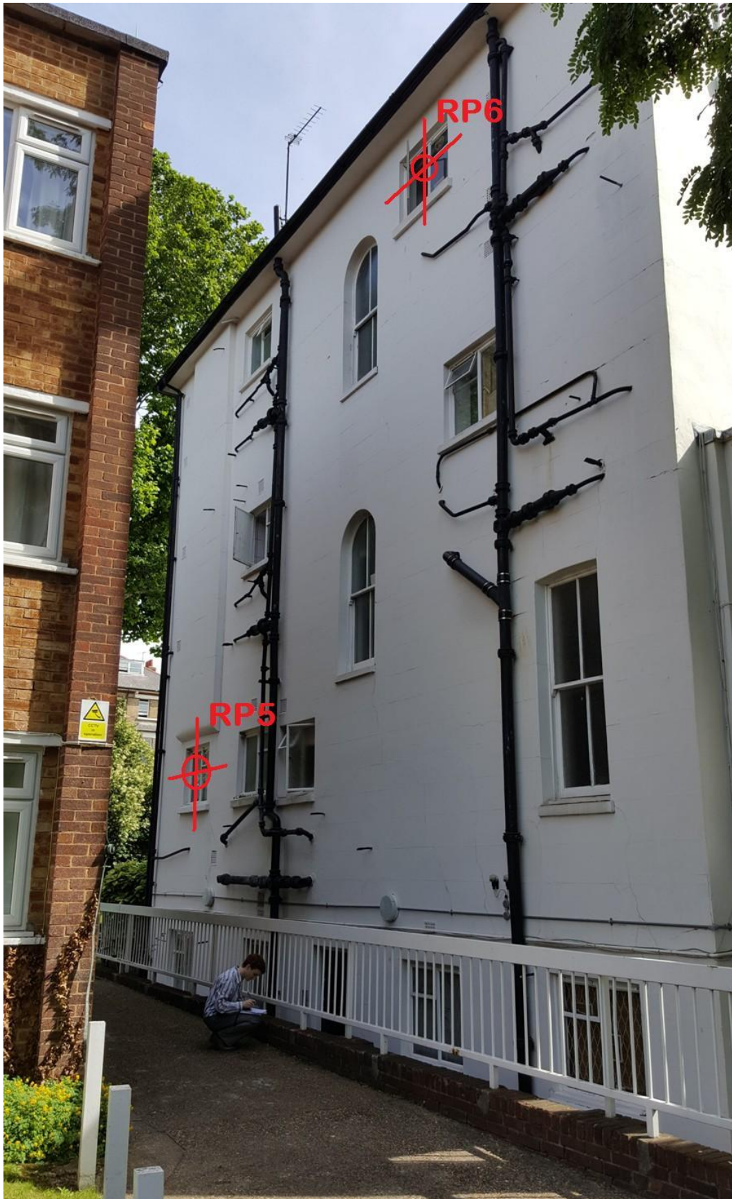
3: Flank elevation of 150 Abbey Road showing locations of kitchen windows
