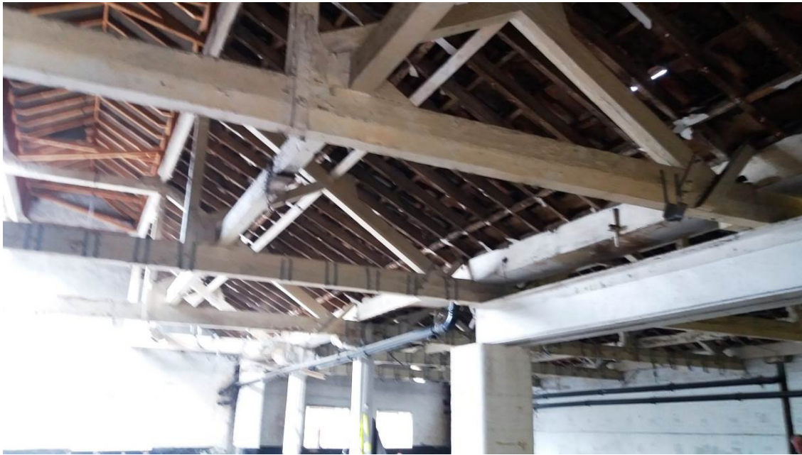
P22 – Existing roof structure supported on steel beam
