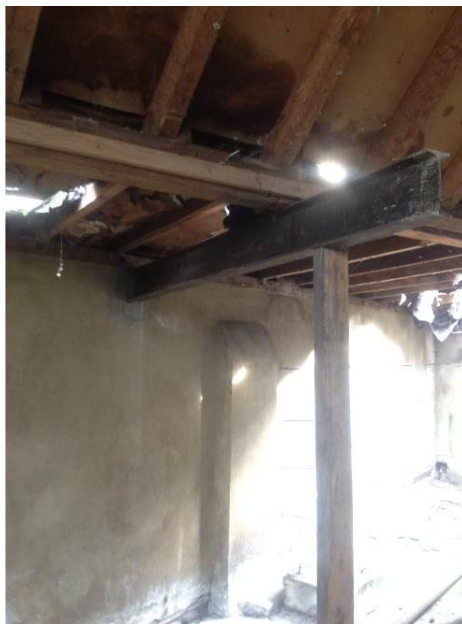
P05 – Remedial steel beam support to collapsing roof
