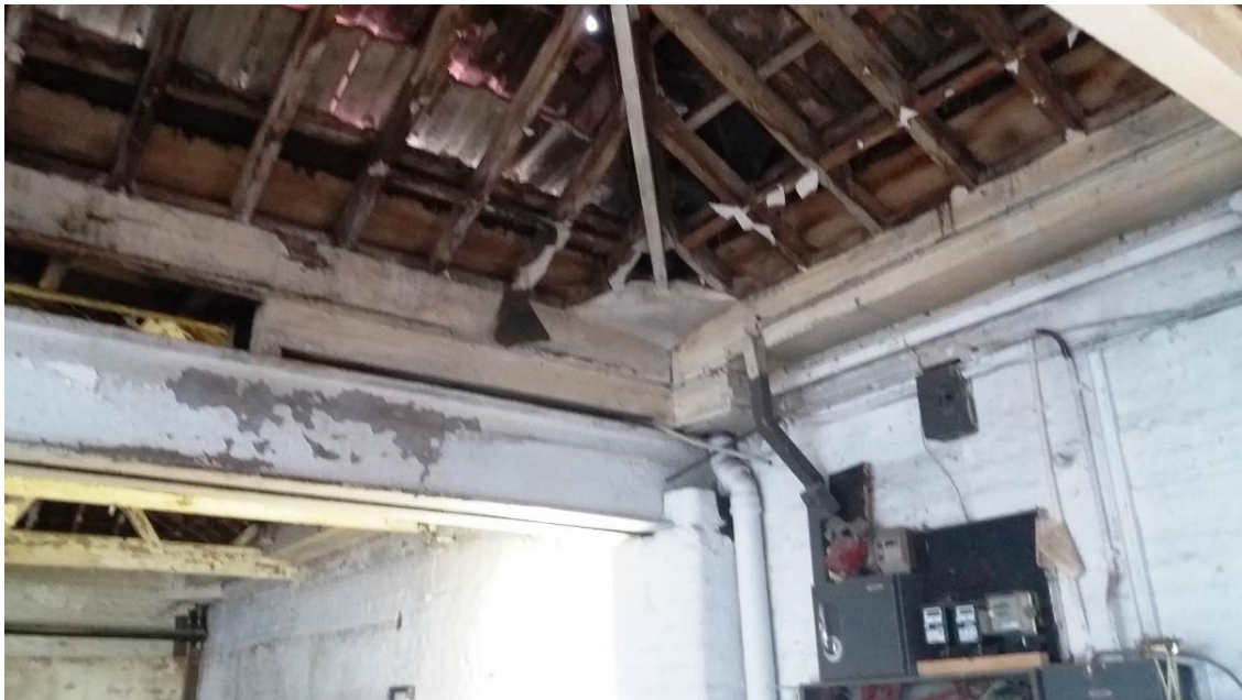
P23 – Existing roof structure supported on steel beam
