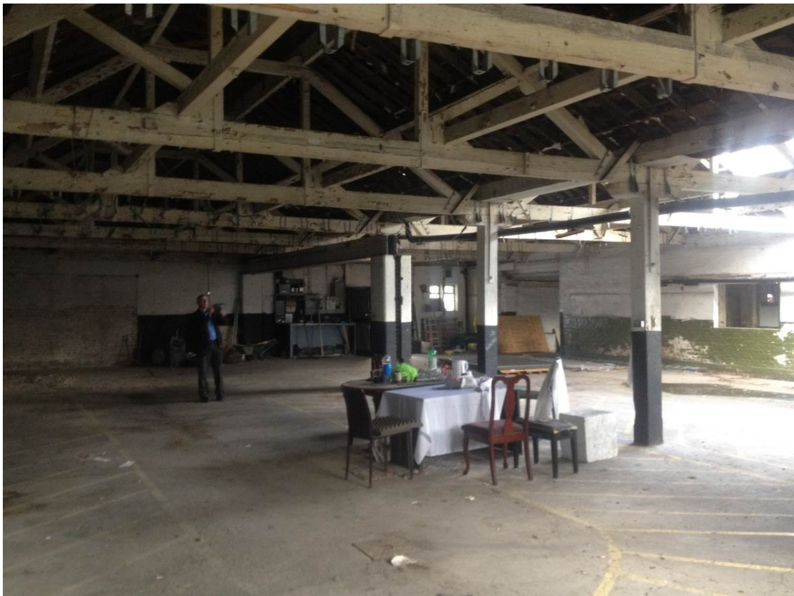
P29 – Internal view of warehouse roof
