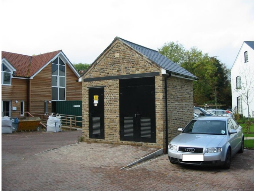
Photo 9: Substation with 'pitched' roof ~ Example 1;
