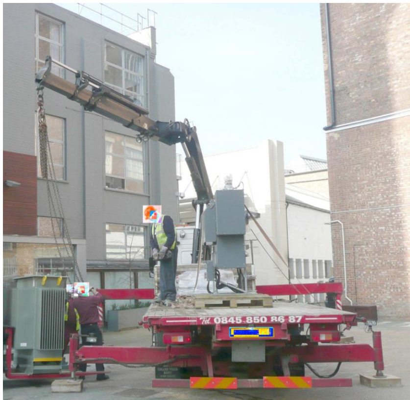
Photo 2: Example of plant delivery with 'out-riggers';
