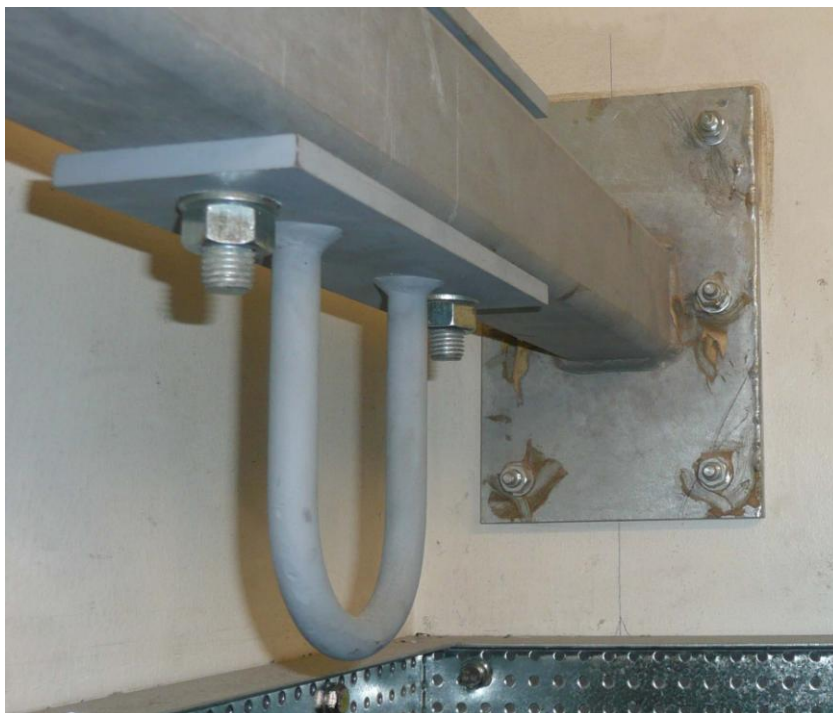
Photo 13: Example of 'Winching eye' for cable installation.
