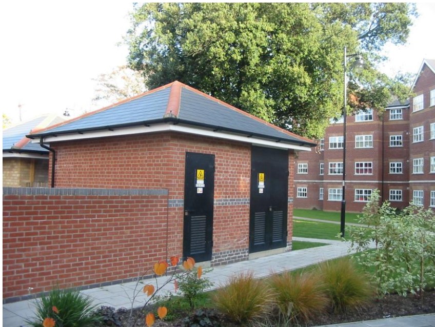
Photo 10: Substation with 'pitched' roof ~ Example 2.
