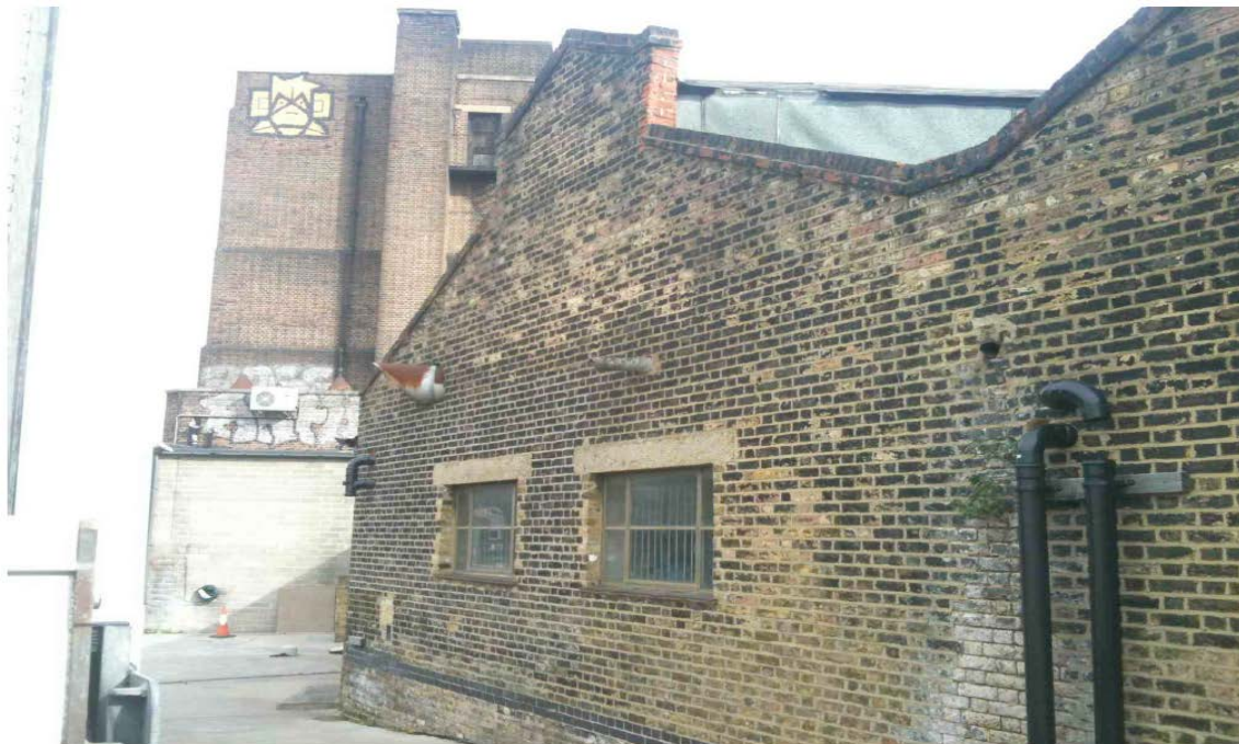
Photograph 2: Rear elevation (south west) of 1A Highgate Road
