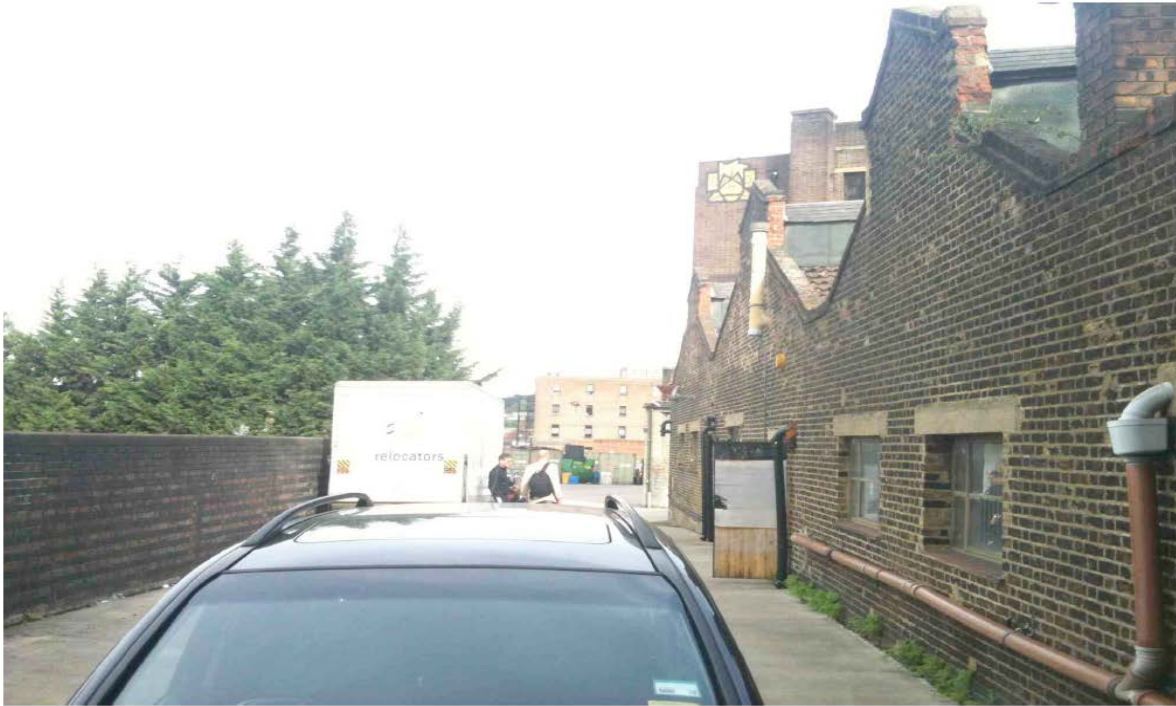
Photograph 3: Rear elevation (south west) of 1A Highgate Road
