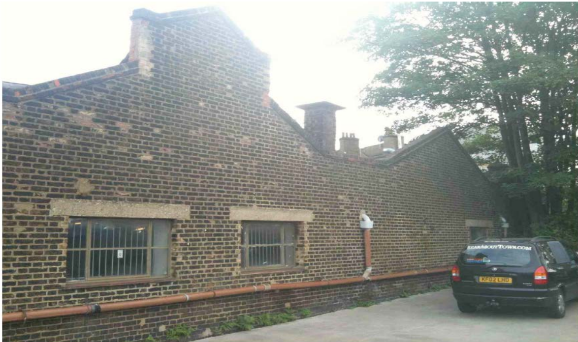
Photograph 5: Rear elevation (south west) of 1A Highgate Road
