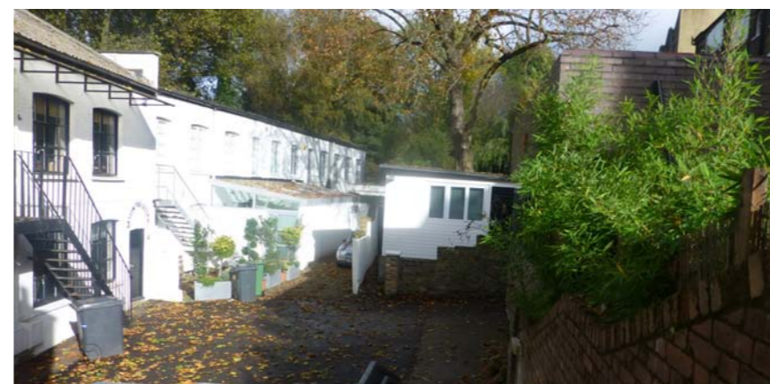
View of shared courtyard looking north
