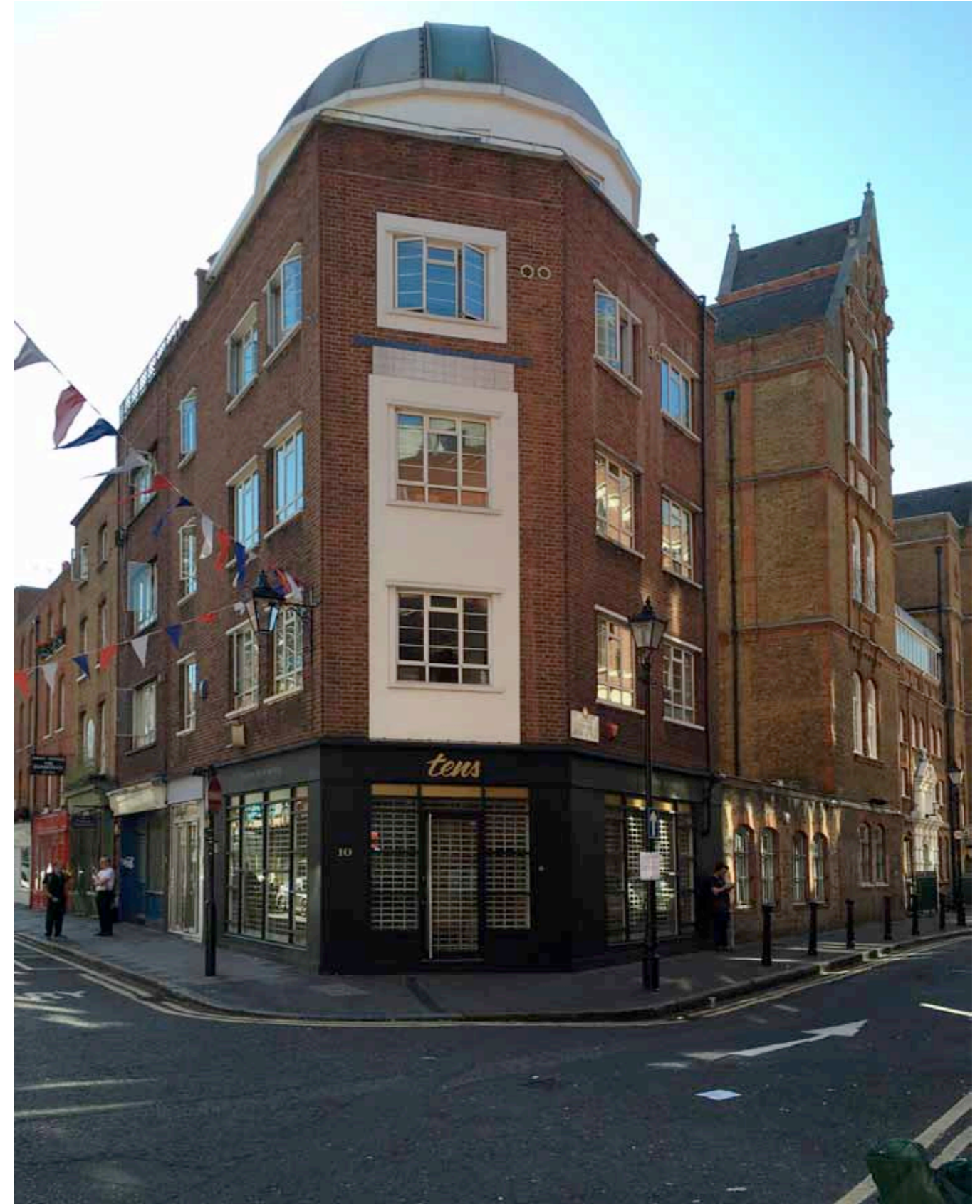
10 and 12 Earlham Street seen from the junction of Earlham Street and Tower Street
