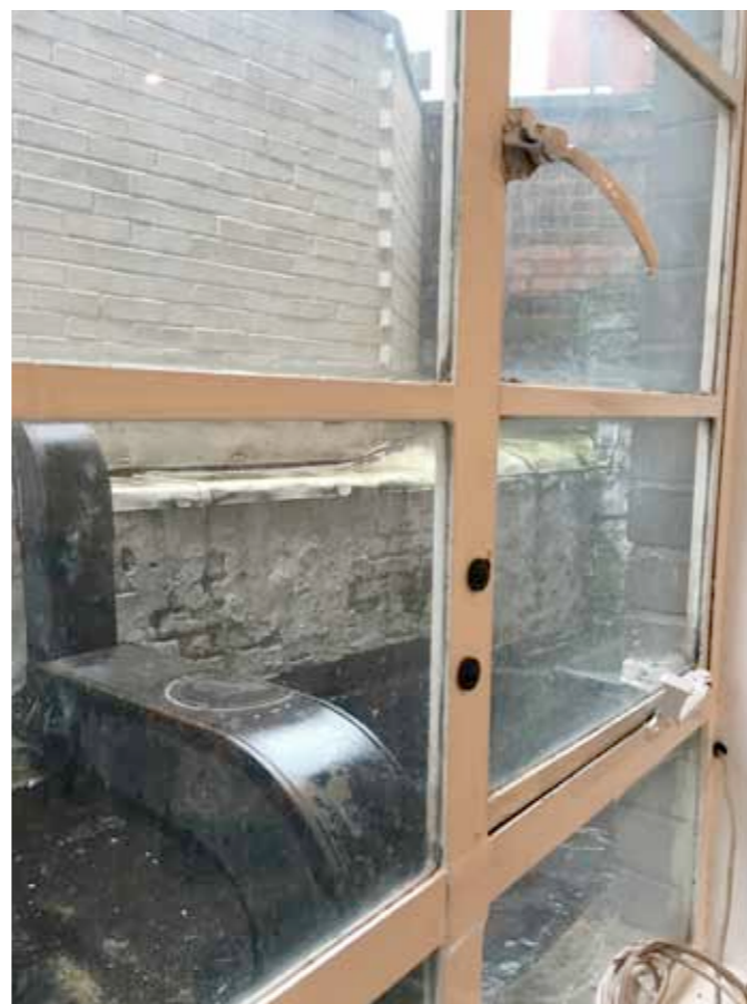
Rear courtyard seen through ground floor window
