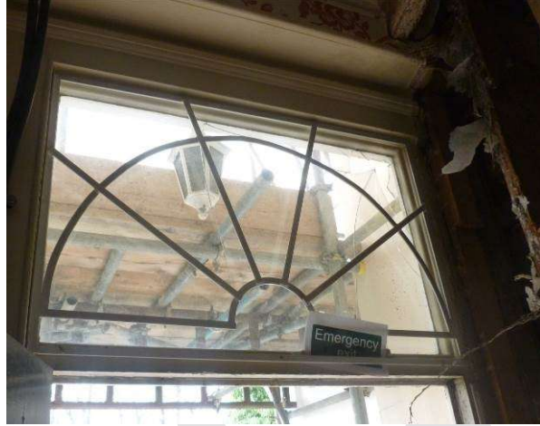
Photo 23: Existing plastic faux fanlight over front door.
