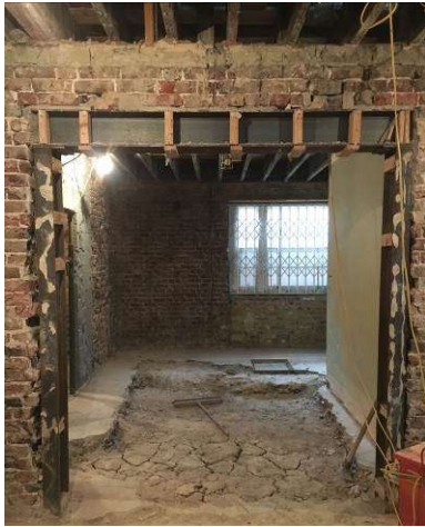
Photo 3: Lower ground floor
