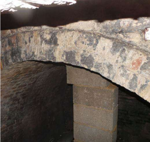
Photo 26: inaccessible vault (seen through hole).
