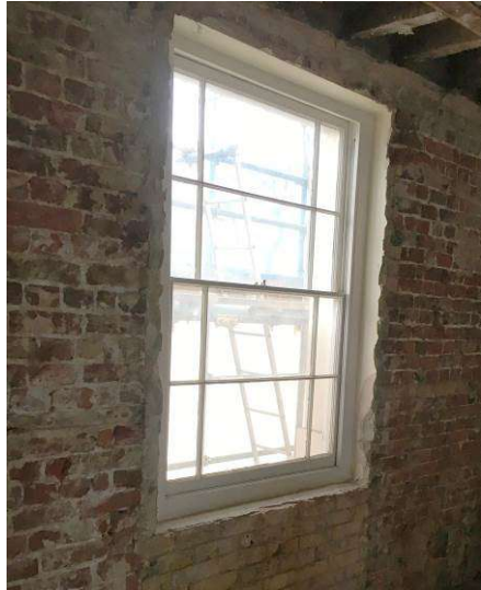
Photo 14: sash window, second floor
