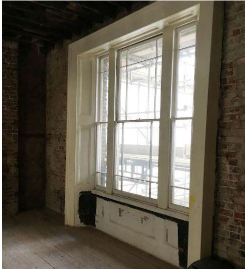
Photo 13: sash window and surround, first floor
