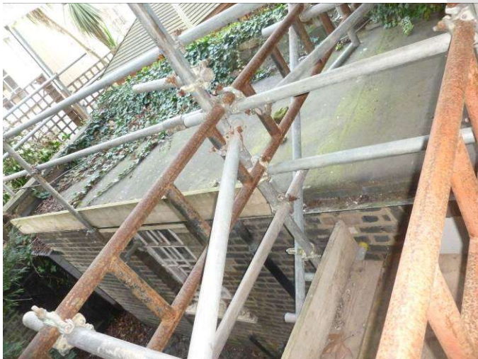
Photo16 : Asphalt roof to rear extension
