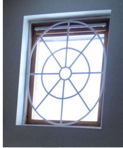
Photo 24: Existing modern rooflight
