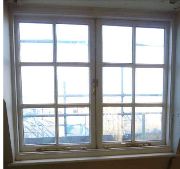
Photo 15: modern double-glazed dormer window third floor
