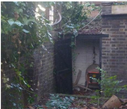
Shed at rear of the site.
