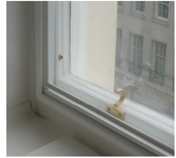
Typical slim secondary glazing added to period sash windows.
