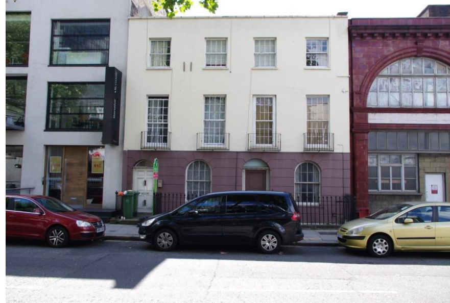
Figure 13: View looking west at the front elevation of the Grade II listed 14-15 Melton Street.
