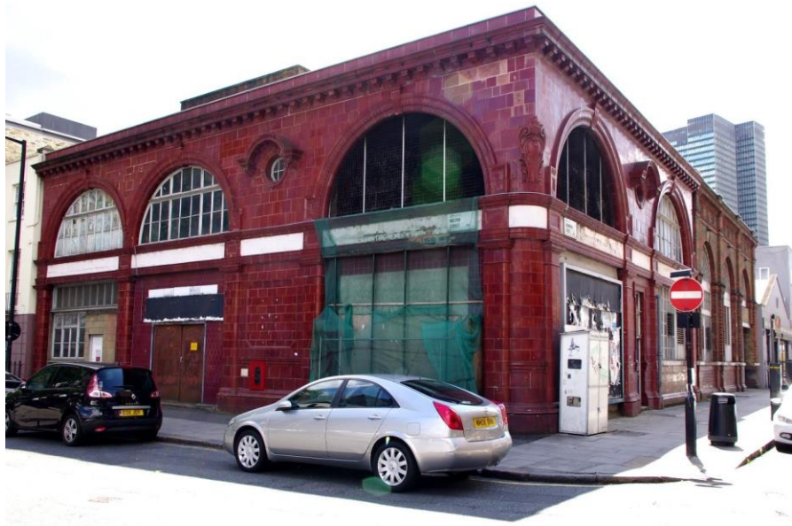
Figure 17: Former CCE&HR underground railway station on the corner of Melton Street and Drummond Street showing the distinctive ox blood faience tiles utilised by Leslie Green at many other London Underground stations.
