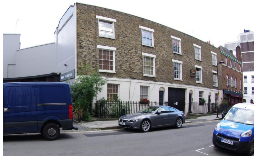
Figure 18: Front elevation of 59-67 Cobourg Street with the Site adjacent (left) presenting a rather intact Georgian terrace row.
