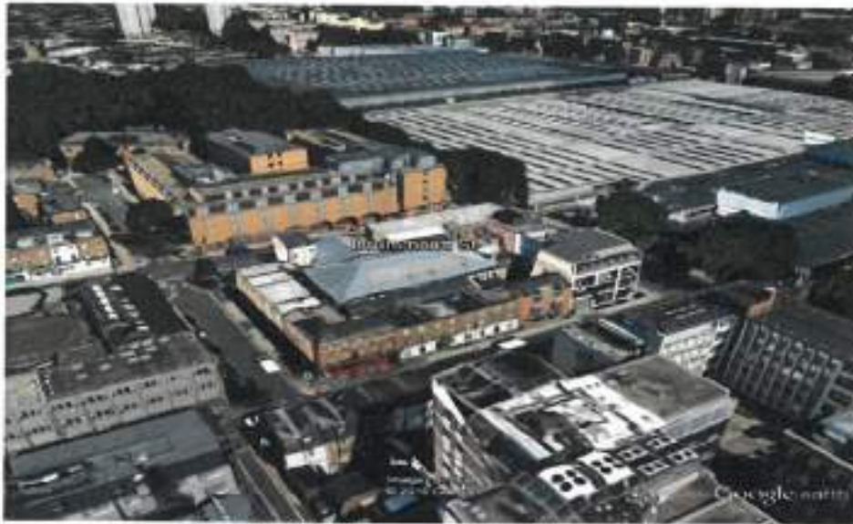
Existing 93-103 Drummond Street Site London.
