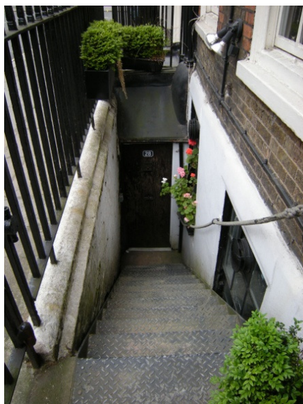
Existing stair and rope handrail
