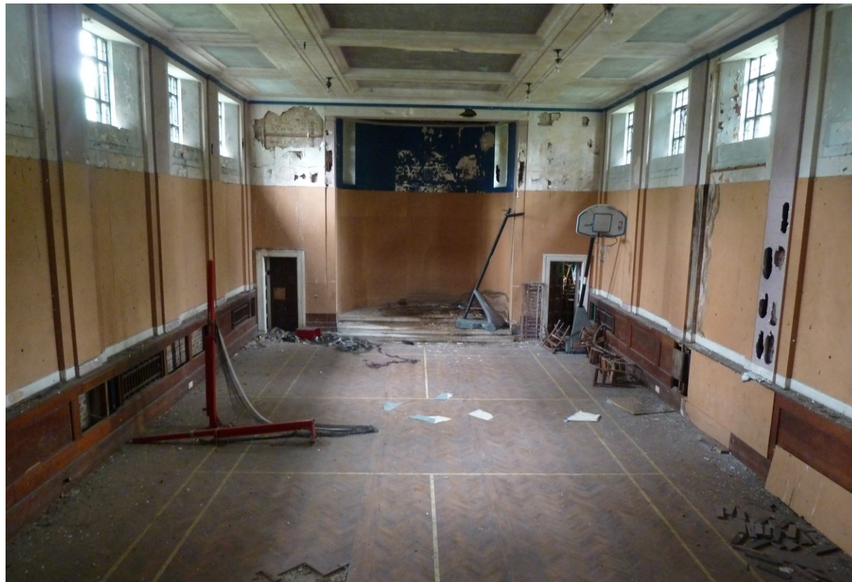
Figure 110. A view of the interior of the Chapel as seen from the entrance from the east elevation.
