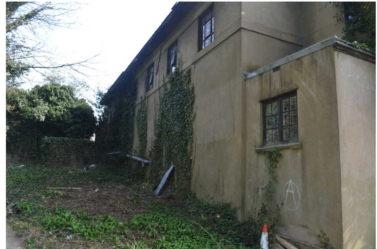
Figure 108. An image of the north elevation of the Chapel which is partially subsumed in the high ground level in this location.
