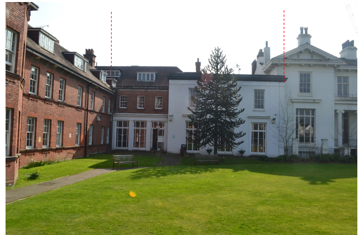
Figure 100 An image of the rear Bay House extension in its context with Kidderpore Hall and the Maynard Wing. The dotted red lines indicate the extent of the Bay House Lounge as seen from the rear from the garden.
