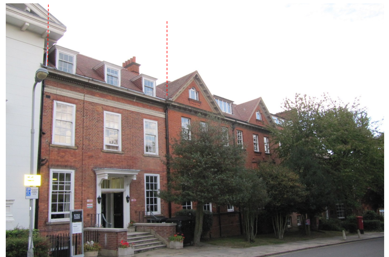
Figure 101. A photograph of the 1921 Bay House extension as seen from Kidderpore Avenue. The red dotted lines are indicative of the extent of the Bay House infill.
