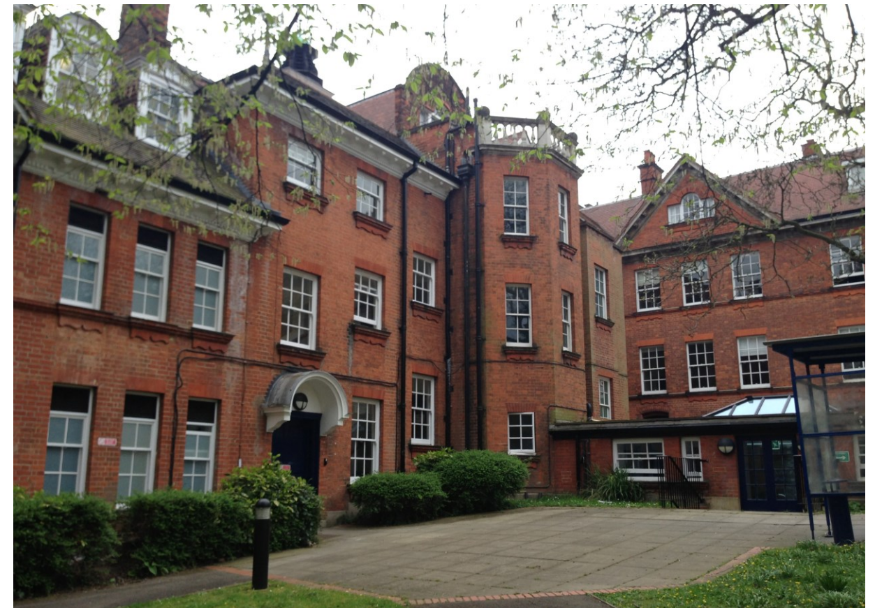
Figure 92. A photograph of the rear elevation of Dudin Brown with the canted bay structure containing the original staircase to the former Skeel Library.
