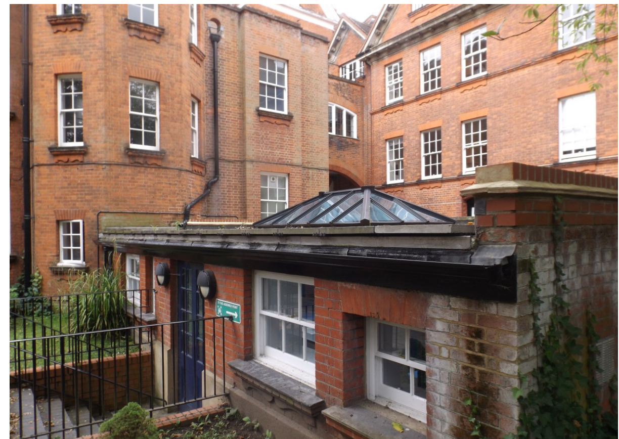
Figure 91. The single storey extension to the rear of the former Skeel Library.
