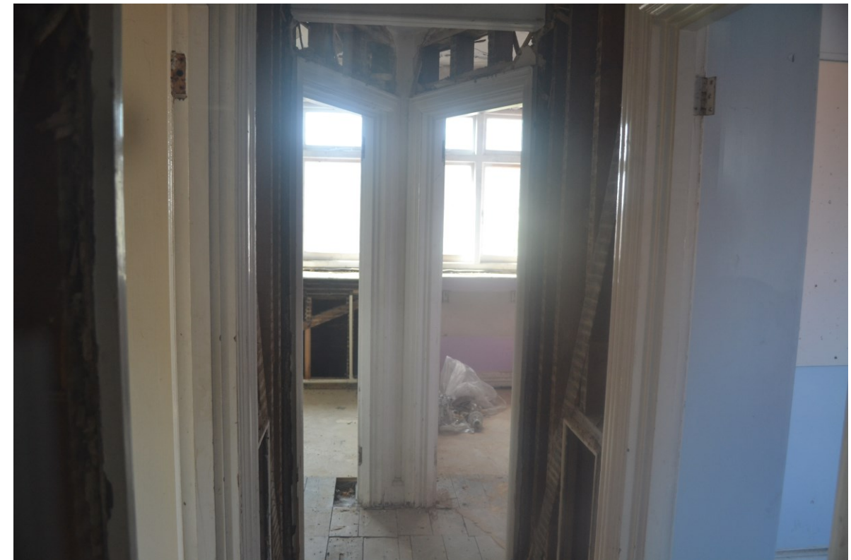
Figure 94. A photograph of the internal partitions at the second floor level.
