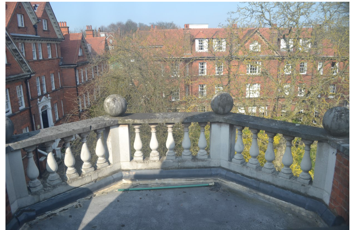
Figure 90. The balcony at the second floor level to the rear of the former Skeel Library.
