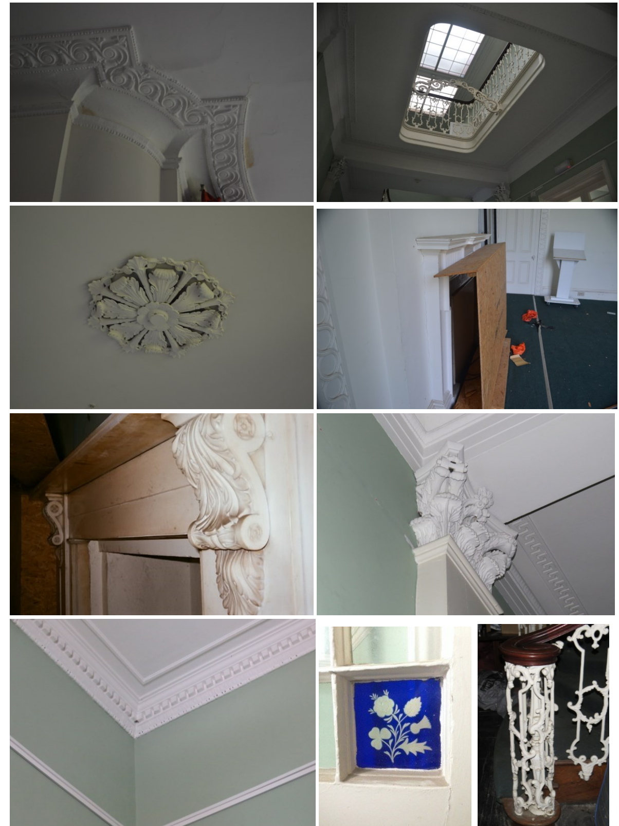
Figure 69. A palette of architectural features which are retained within Kidderpore Hall at the ground and first floor levels. Most of these features, including the balustrades to the principal staircase, the cornice and ceiling roses are original to the property.
