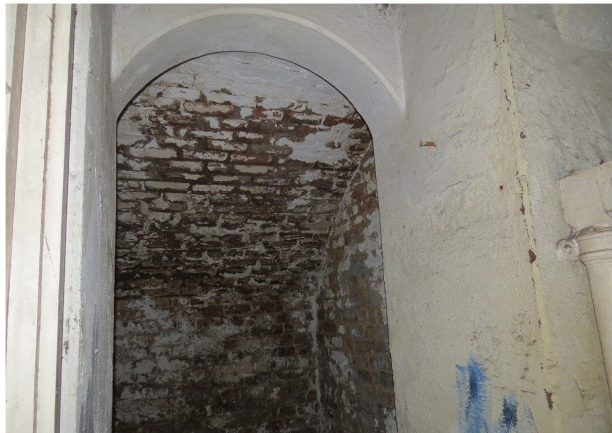
Figure 64. A photograph of one of the vaults at the basement level of Kidderpore Hall located underneath the pavement.
