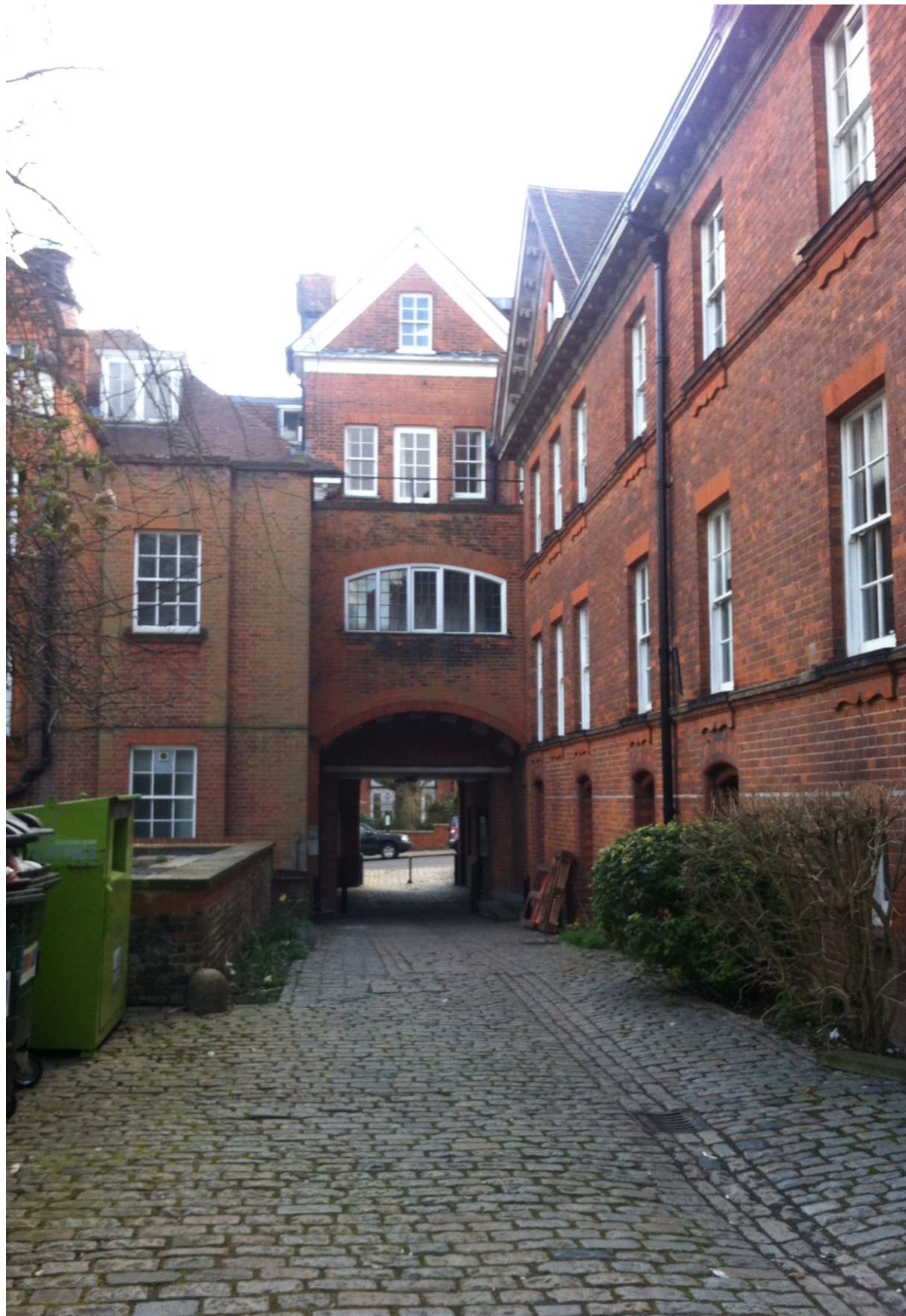
Figure 78 A photograph of the cobbled walkway to the east of Maynard wing looking towards Kidderpore Avenue.
