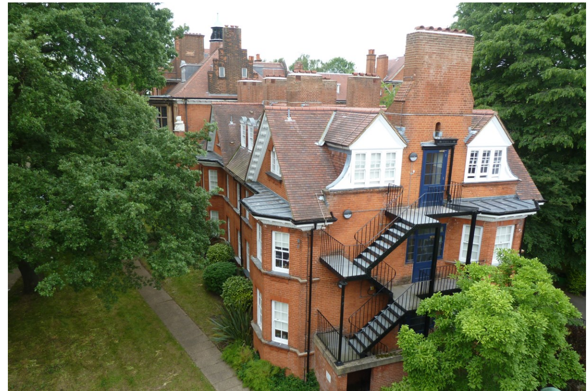
Figure 33 An aerial view showing the later addition of the fire escape staircase.
