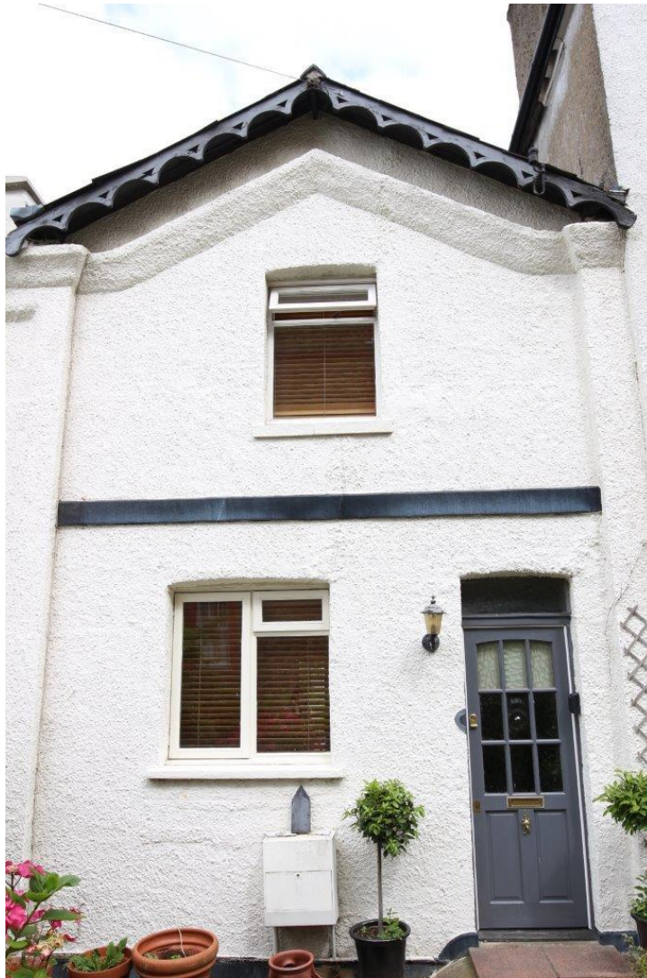
1. No. 8 West Cottages front elevation
