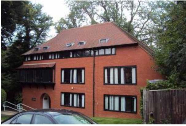
Photo 1 – Existing Queen Mother Hall
