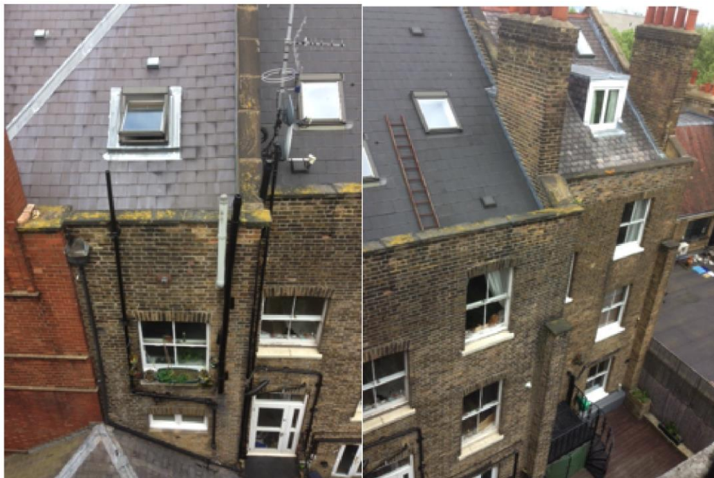
Fig. 8 Photos showing existing view from roof level to neighbouring windows of Nos. 65-67 Hampstead High Street
