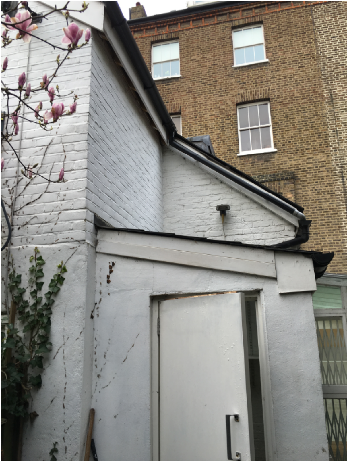
Photograph3: Facing adjoining neighbouring property 'The Studio' on No.76 Parkhill Road.
