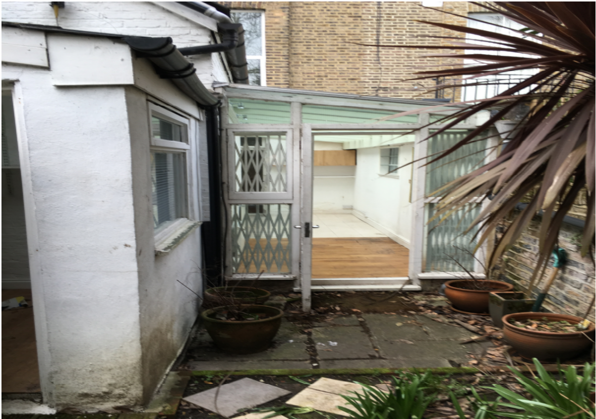
Photograph 1: Existing conservatory and location of proposed extension
