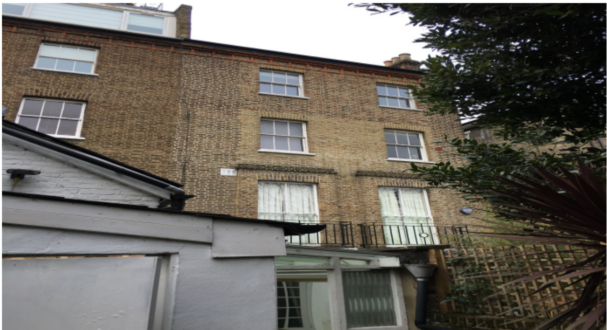
Photograph 2: Proposal area and facing towards adjoining neighbour No.78 Parkhill
