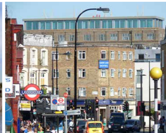
Belmont Street warehouse conversion and roof extension
