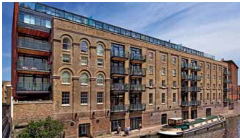
The Henson Building, Camden Town
