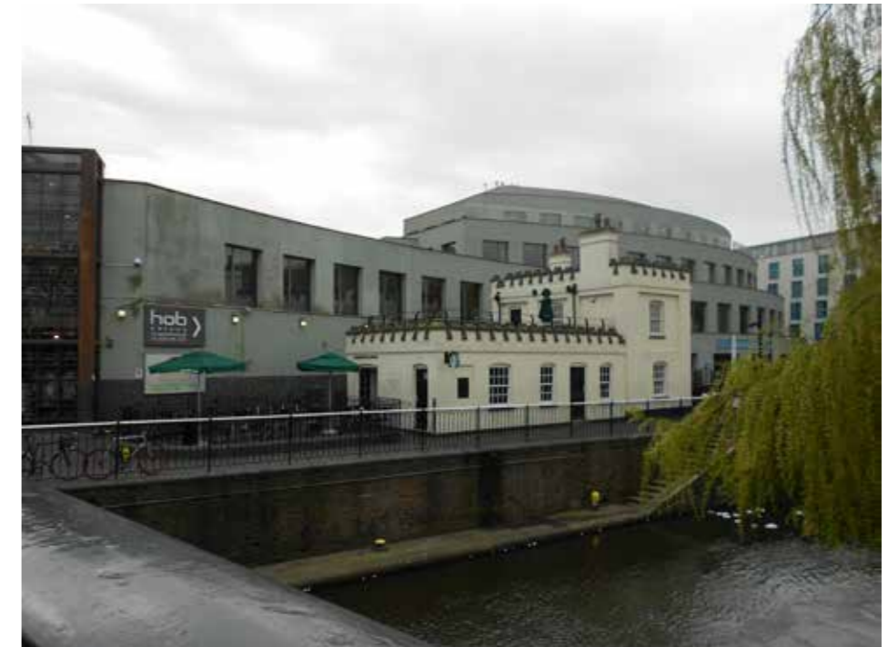
1. Existing Photo from Chalk Farm Road on Hampstead bridge
