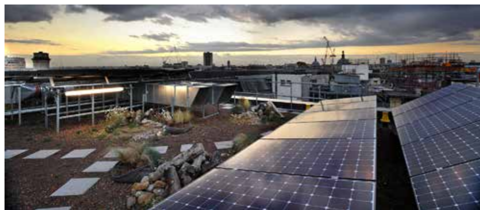
PV panels and green roof combined
