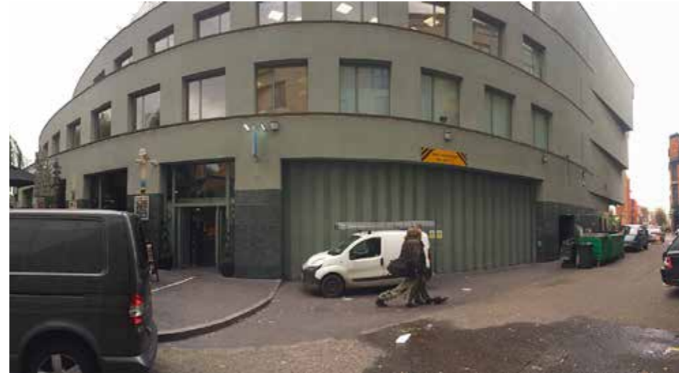
View of existing service yard entrance
