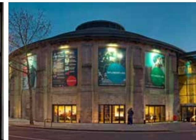
The Roundhouse Refurbishment
