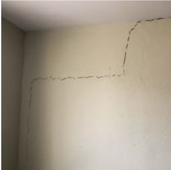
11. Internal Partition Cracking At Third Floor.
