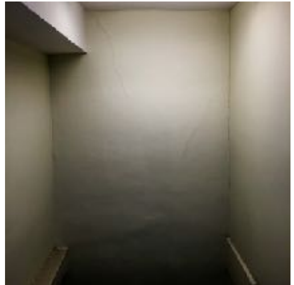
12. View of Cracks In Party Wall At Third Floor.
