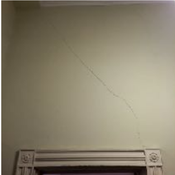
16. View Of Crack In Wall At First Floor.
