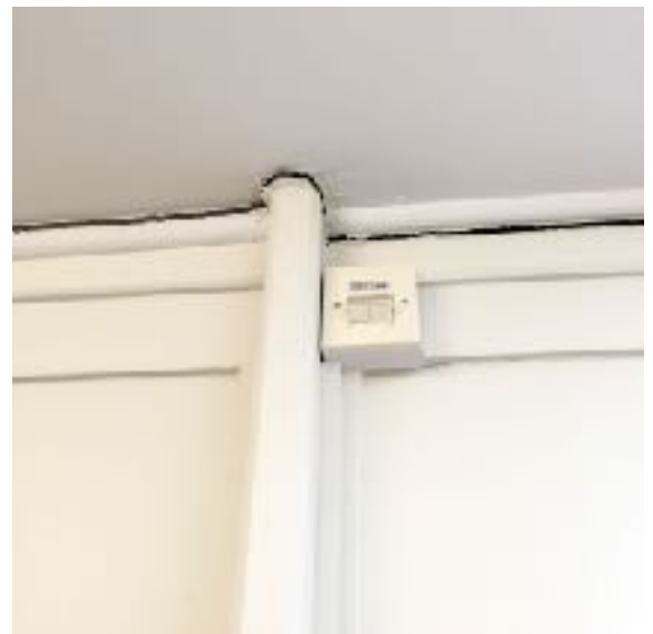
10. View of Corridor Wall Cracking At Third Floor.
