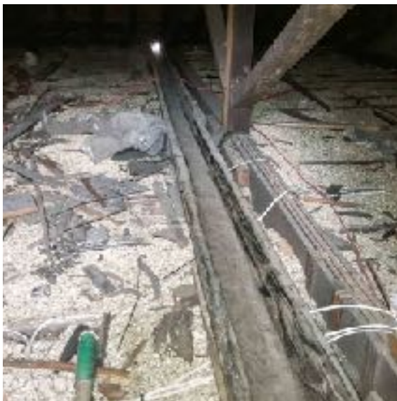
9. View of Internal Open Channel Rainwater Gutter.
