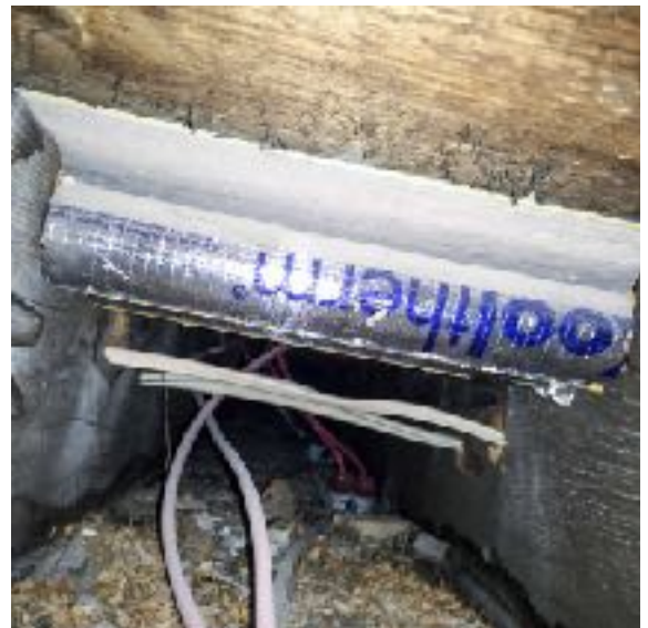
13. View Showing Notched Joists in Third Floor.
