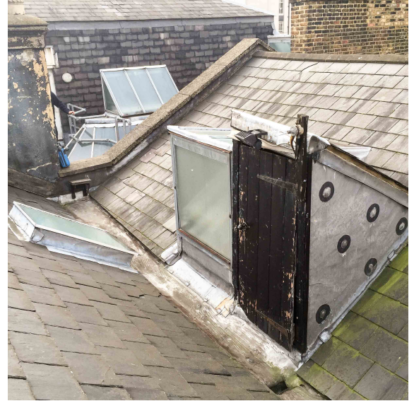
Image 3, View of Roof.
