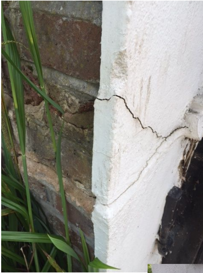
3) and 4) closer views of the cracking visible in photo 2.
