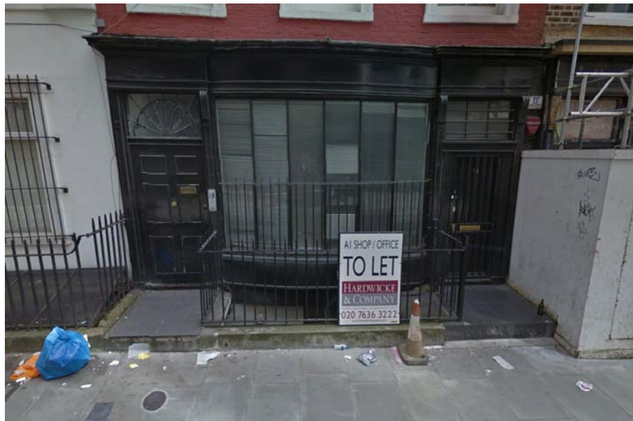
Above: Shopfront of no. 18 Cleveland Street with the residential entrance to the left and the ground floor entrance to the right. Showing bow window with additional security railing and front lightwell with access to the lower ground floor.
