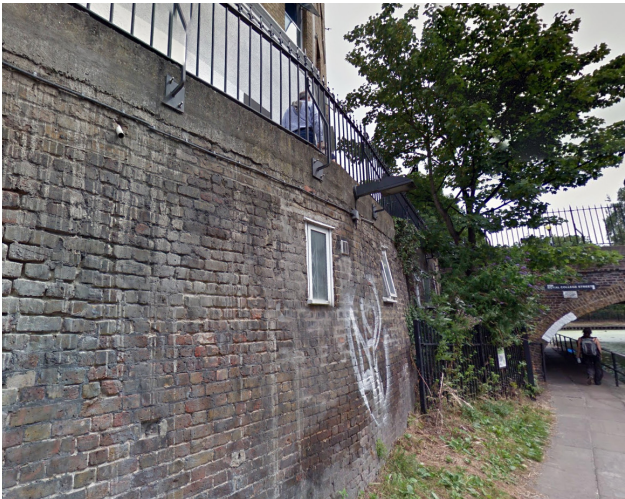
03. View from Regen't Canal Footpath
