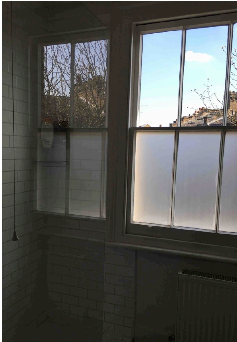
Fig 13. View of existing Shower Room on First floor half landing
