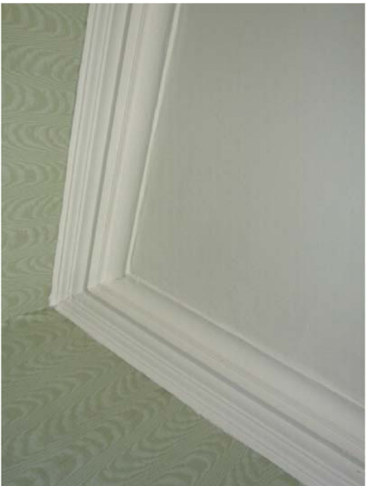
Existing ceiling and cornice to be retained and repaired.
