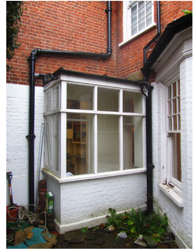
Existing rear extension
