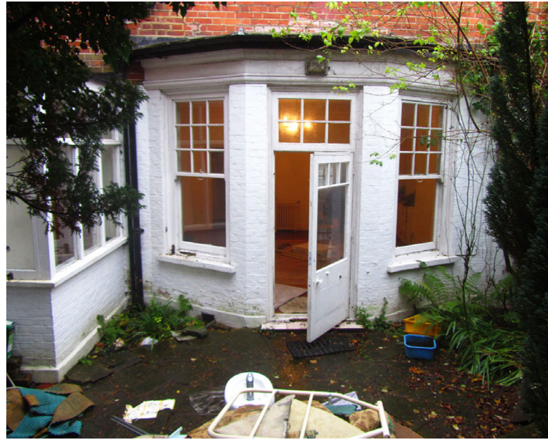
Existing rear elevation, facing Southwest
