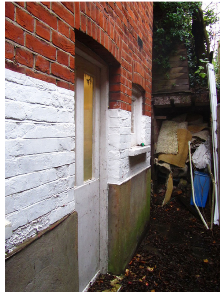
Existing passageway, kitchen door
