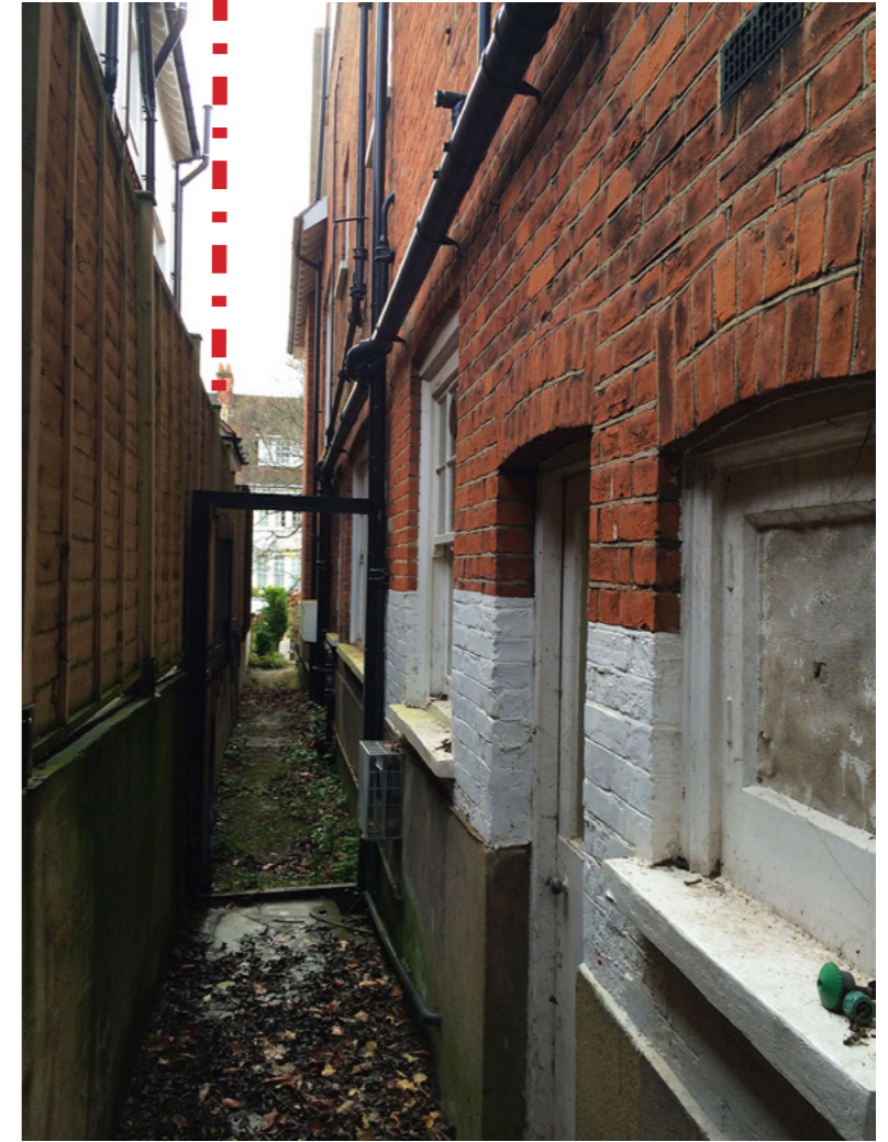
Existing passageway, facing Southeast No. 16 ■ No. 14
