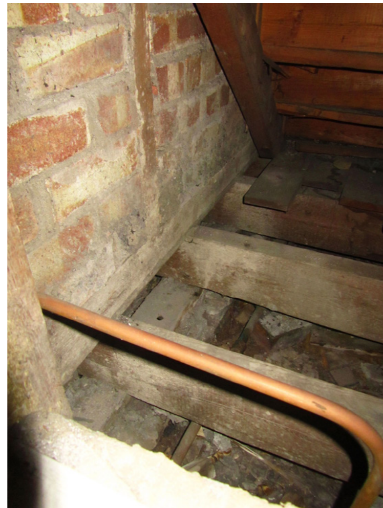
Wall to master bedroom and floor joists beneath the stairs
