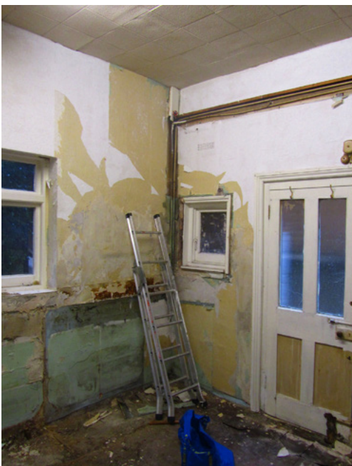
The existing state of the kitchen.
